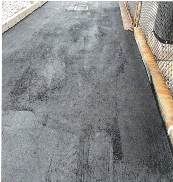
Asphalt Repair pictures at Valley Station
