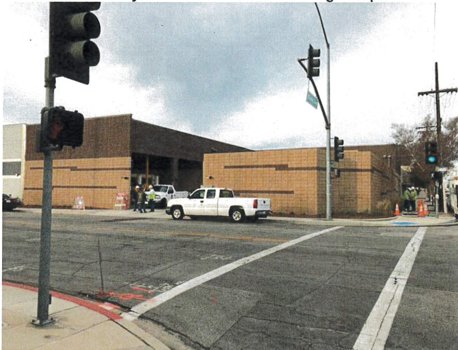
Ontario Substation - Landscaping Complete
