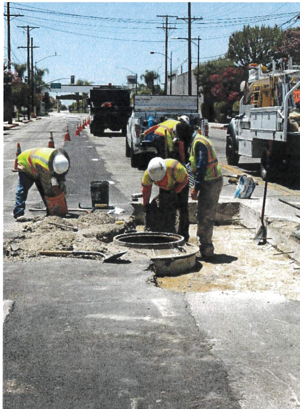
Repaving: MH-630 On Winona Ave.
