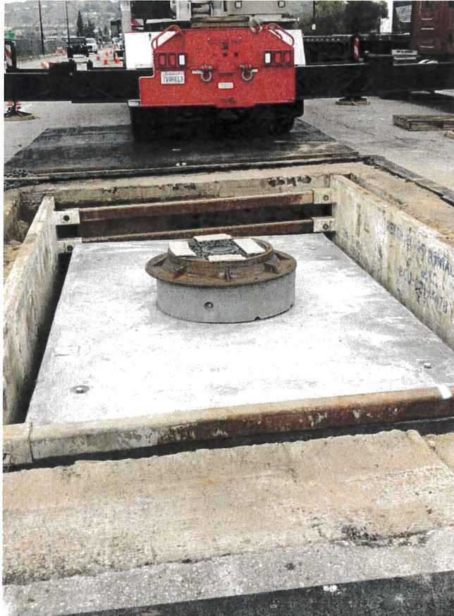
Manhole Installation: Lid installed
