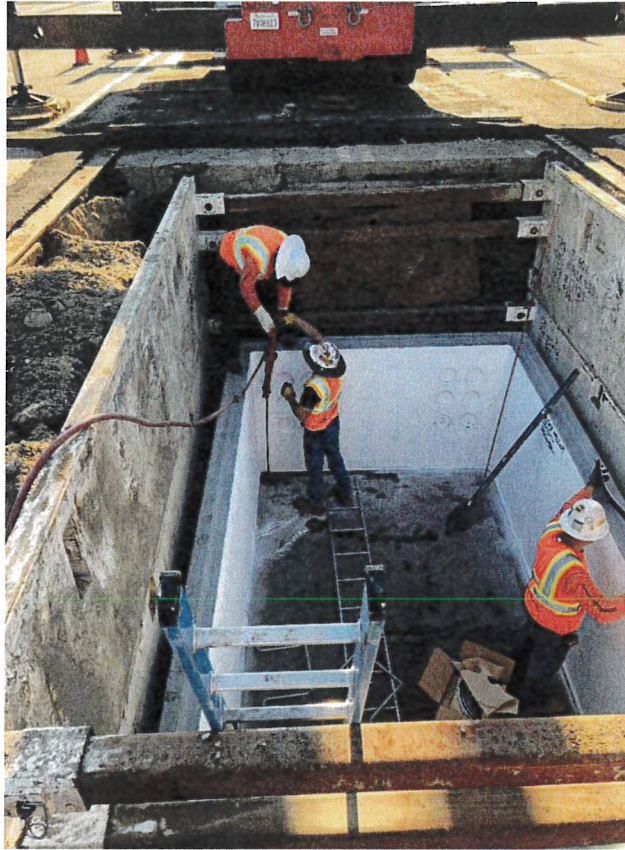
Manhole Installation: Ground rod installation
