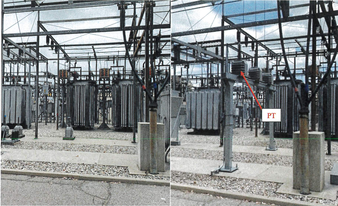
Before PT Installation
