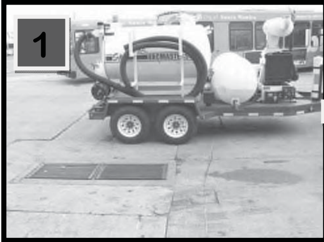
Remove grates from catch basins to gain access to the GISB filters. Special hooks are available from various manufacturers which are designed to remove the grates.
