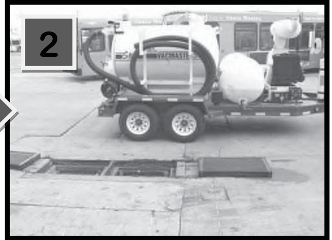
Remove grates from catch basins to gain access to the GISB filters. Special hooks are available from various manufacturers which are designed to remove the grates.
