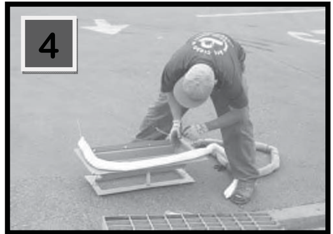
Remove old media boom by cutting zip ties. Replace with new media boom and fasten with zip ties.
