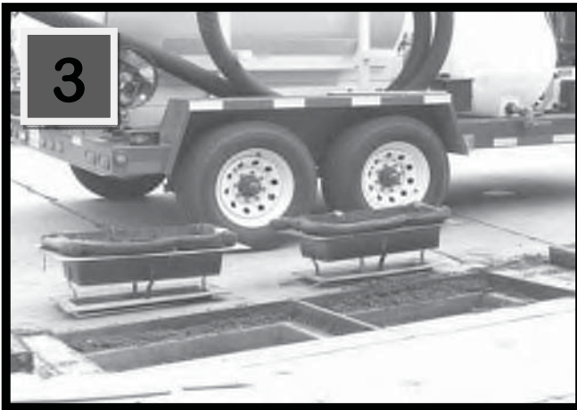
Remove skimmer tray and attached media booms.
