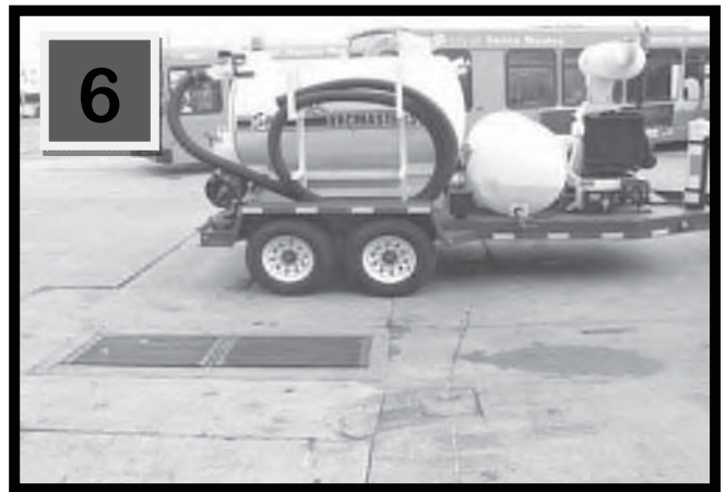
Replace grates. Make sure they are properly re-installed.
