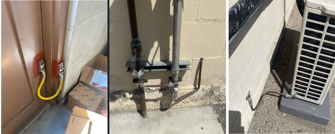
Ground Grid Improvements
