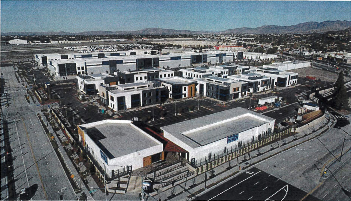
Figure 1 – Aerial photograph looking north-west from Hollywood Way/Tulare (this is Phase 2 of Avion)
