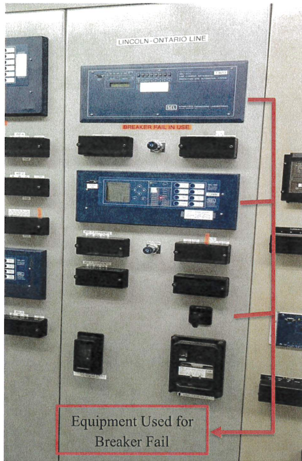
4527 Breaker Fail Addition @ Lincoln Substation
