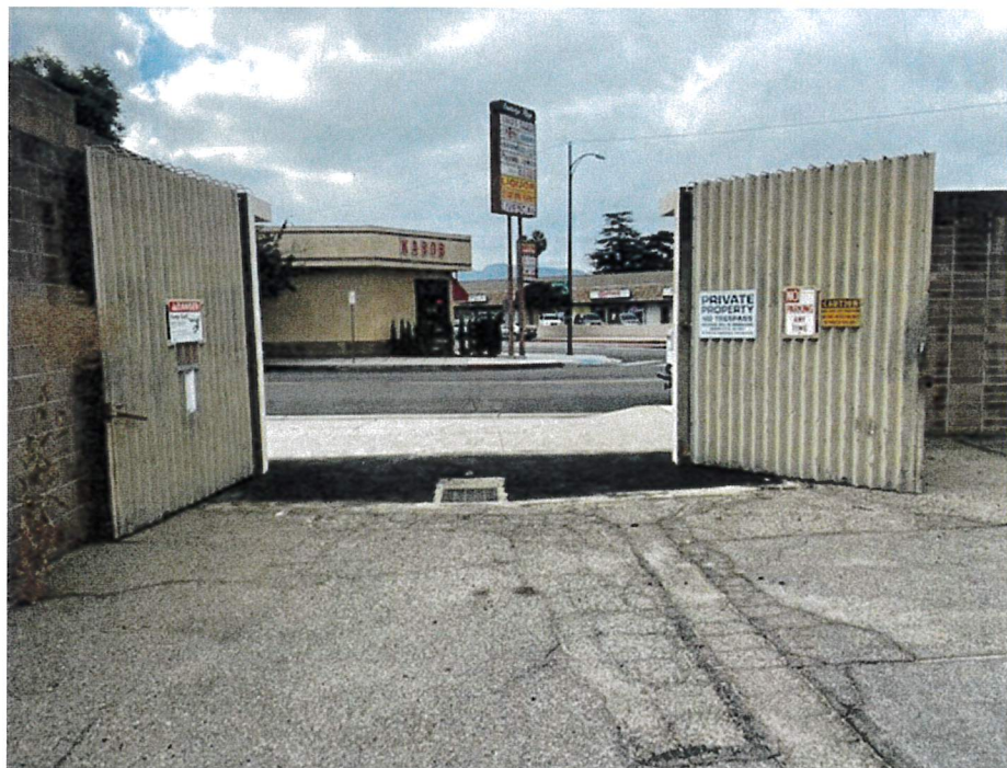
Asphalt Addition Work at McCambridge Substation
