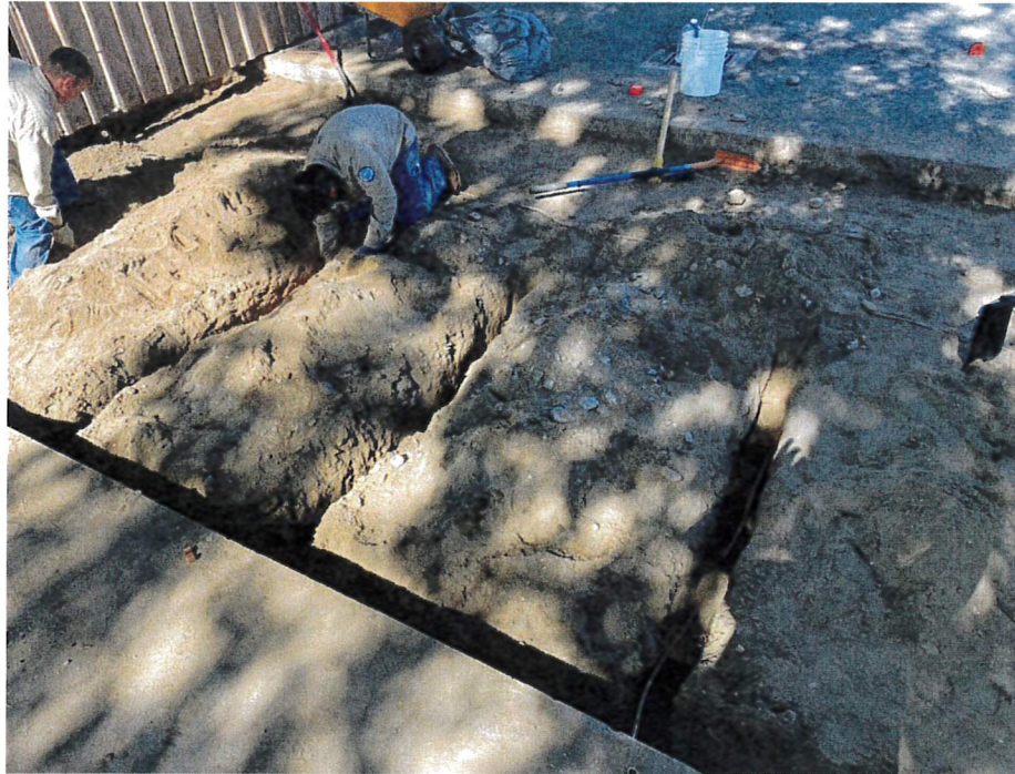
Ground Grid Work at Victory Substation
