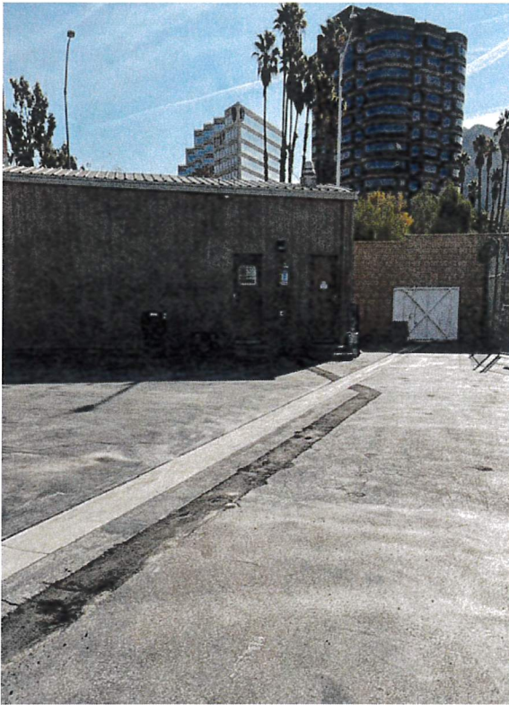
Conduit Trench to Safety Shower
