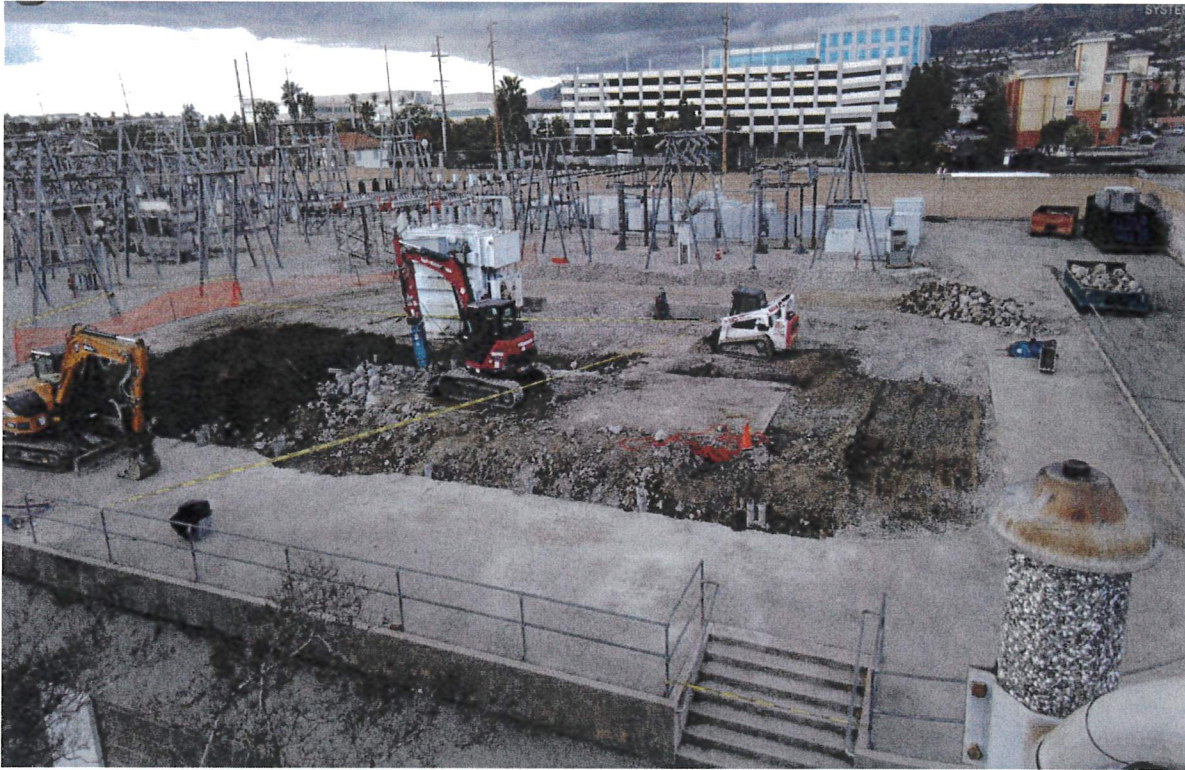
Golden State Substation with most equipment removed
