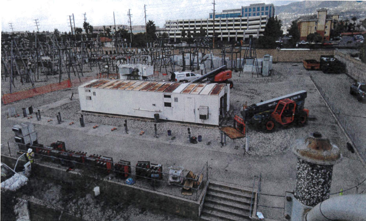
Golden State Substation prior to the demolition
