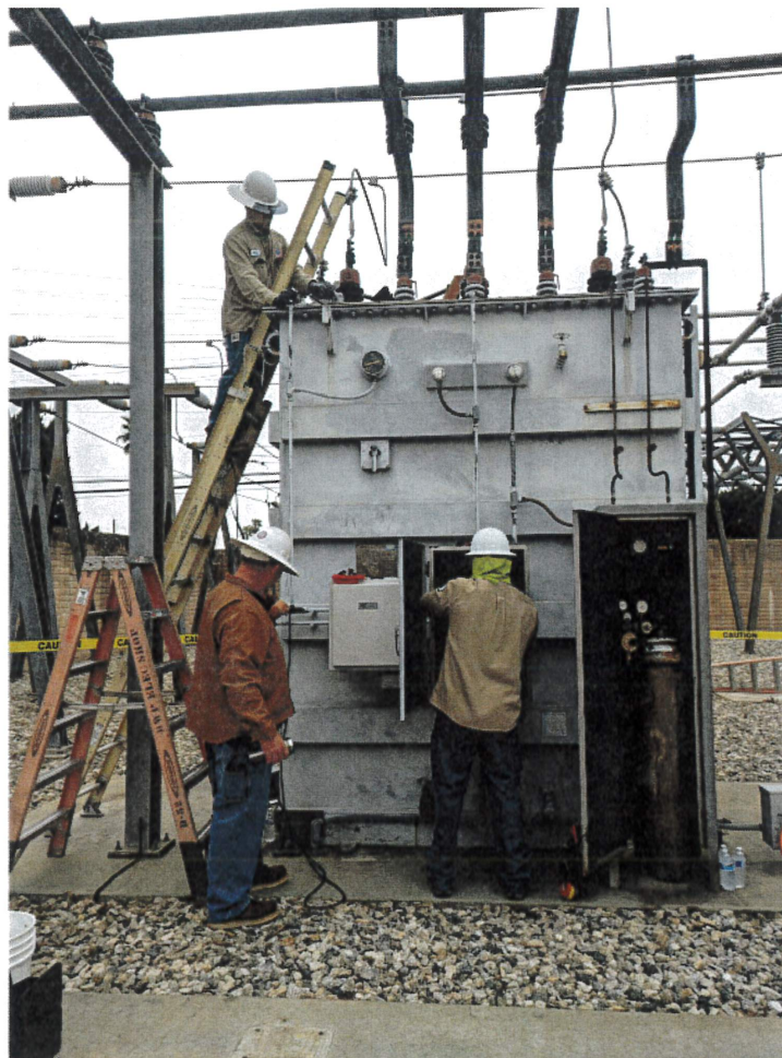
Clybourn A1 Transformer Relay Replacement During Construction
