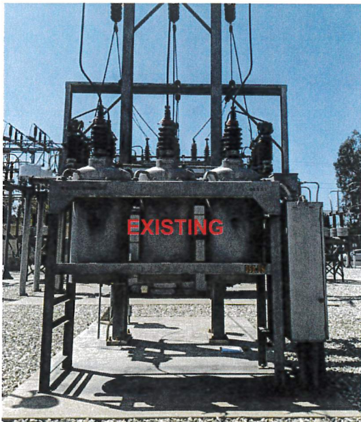
Original 34kV Oil Circuit Breaker at Valley Bk. A-1
