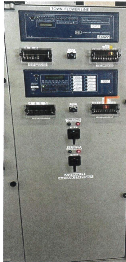
Post Replacement (New Relays)
