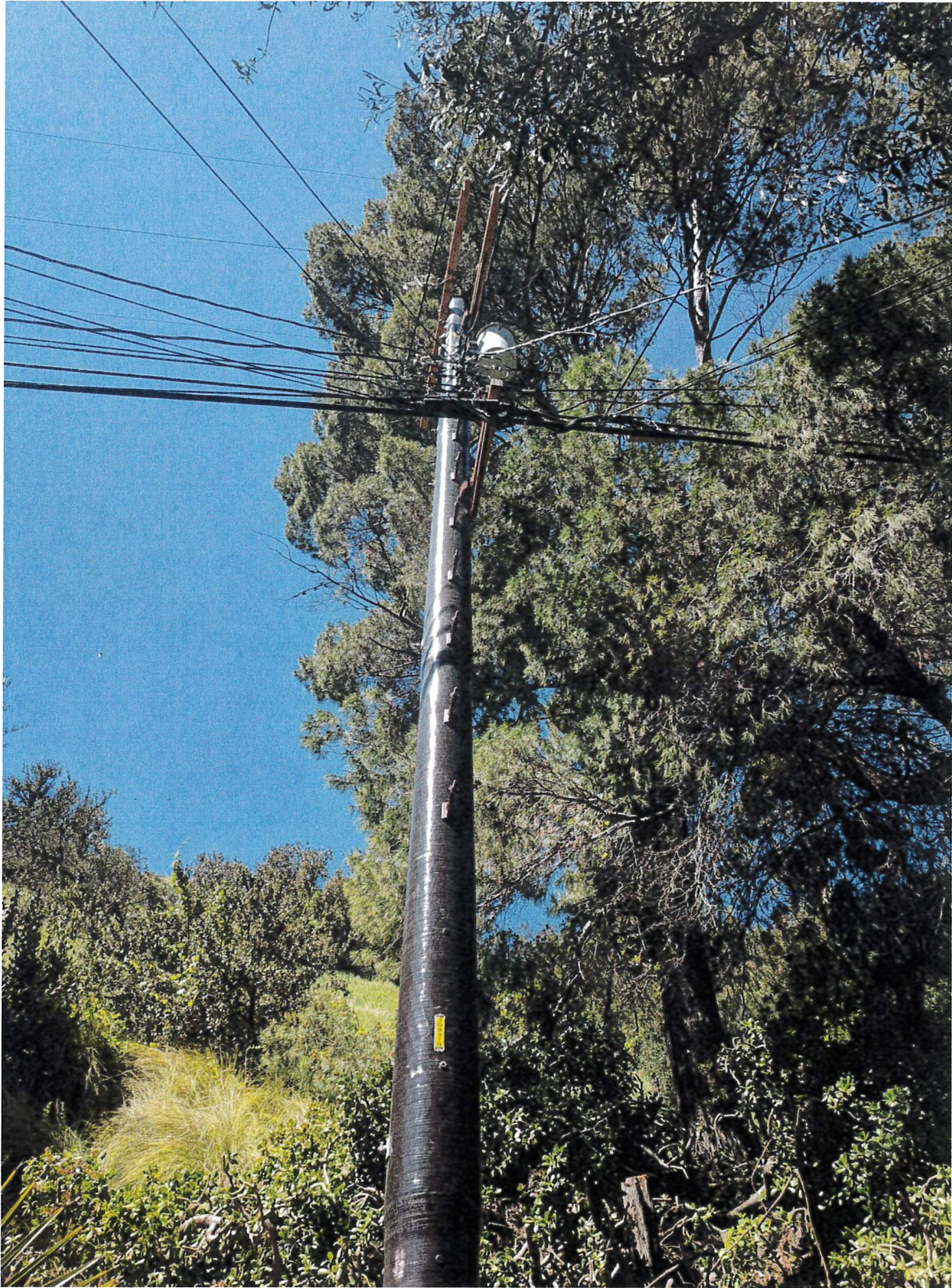
Composite Pole Installed
