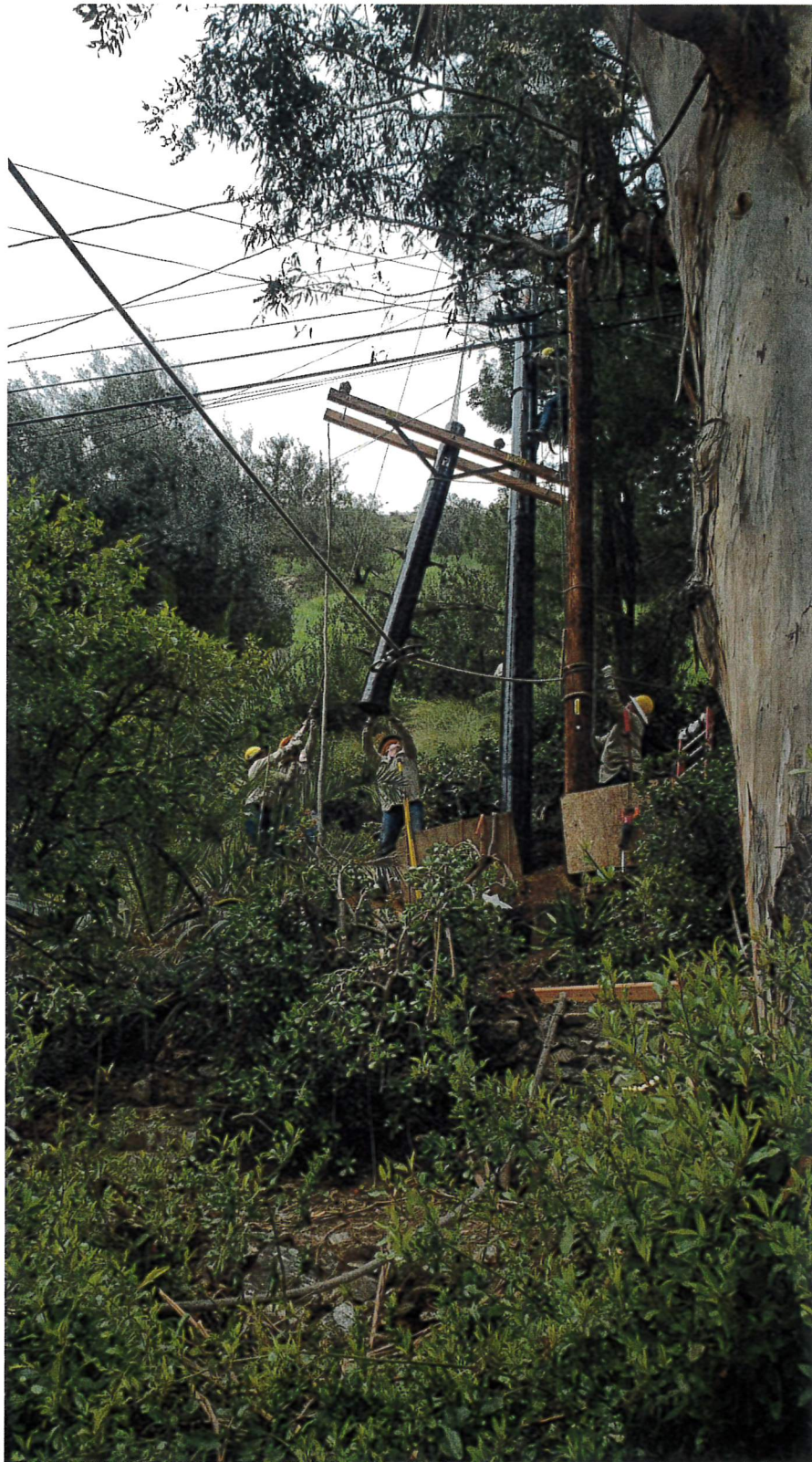
Composite Pole Installation
