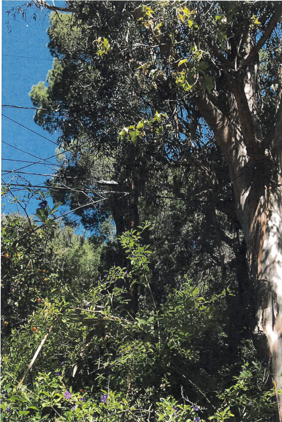
Original Wood Pole in Difficult-to-Reach Location
