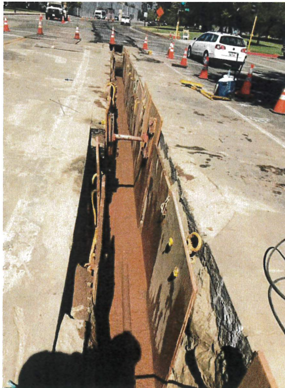
Underground trench for electric conduit installation
