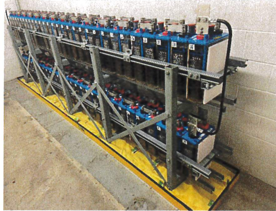
Battery Bank - Installation
