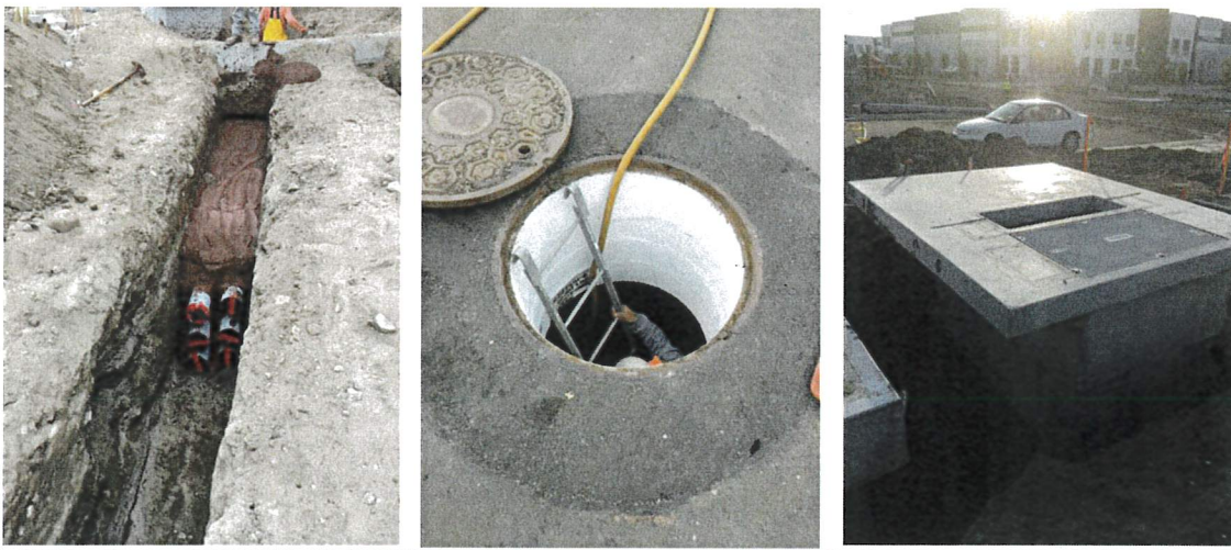
Figure 2 - Underground electrical substructure installations on the project site
