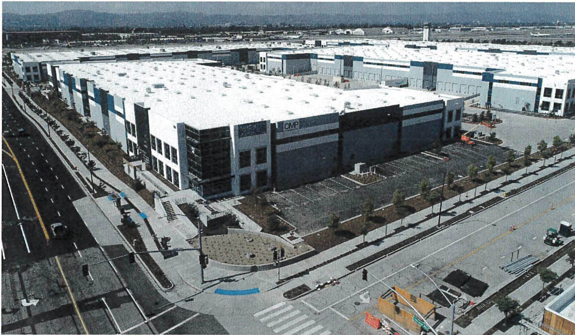
Figure 1 – Aerial photograph looking south-west from Hollywood Way/Tulare (this is phase 1 of Avion)
