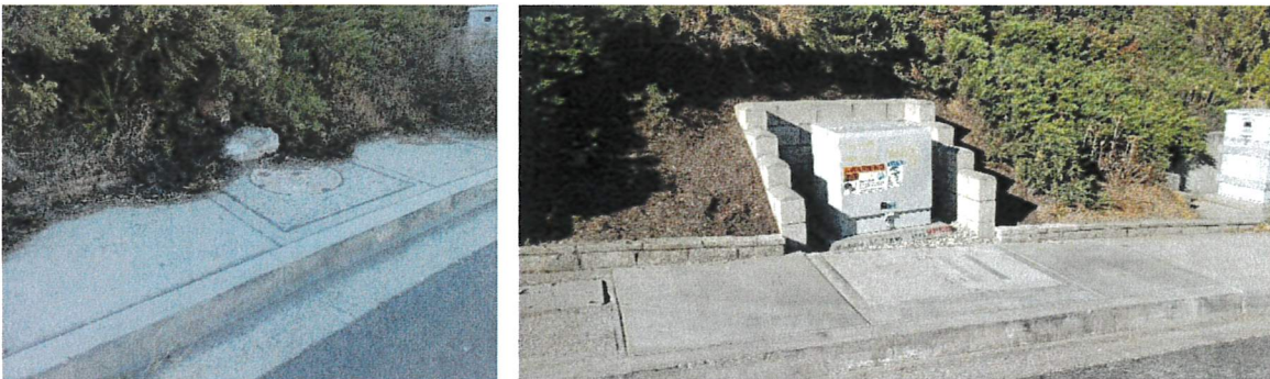
Vault 15 before and after
