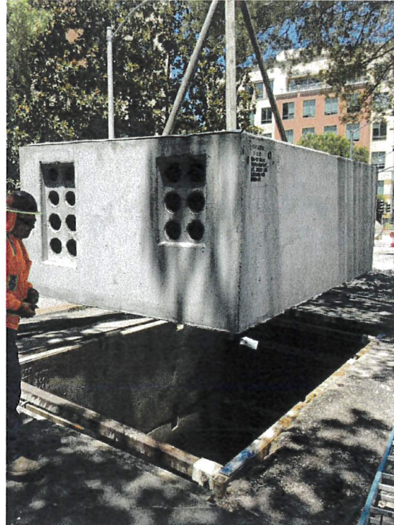
Manhole installation on California St.
