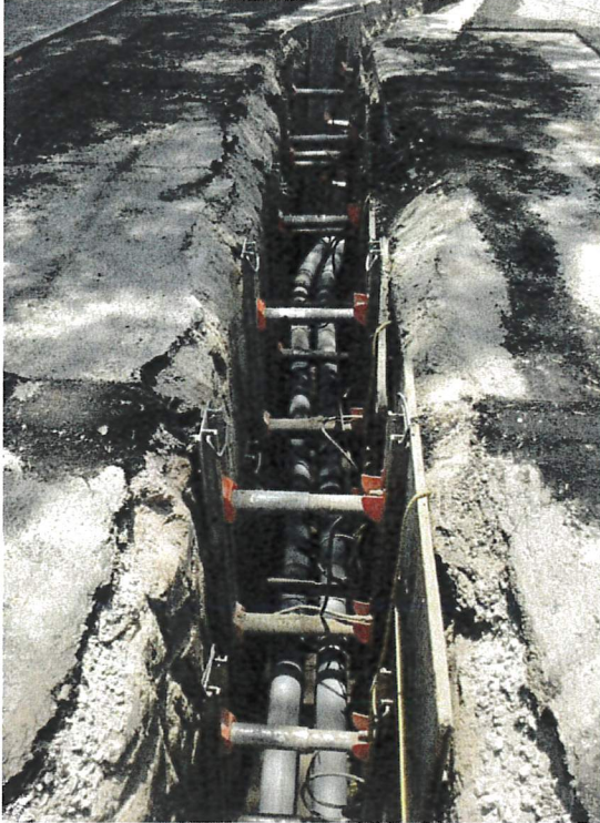
Conduit installation on California St.
