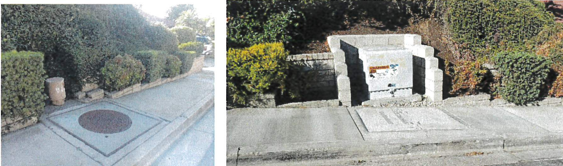
Vault 14 before and after
