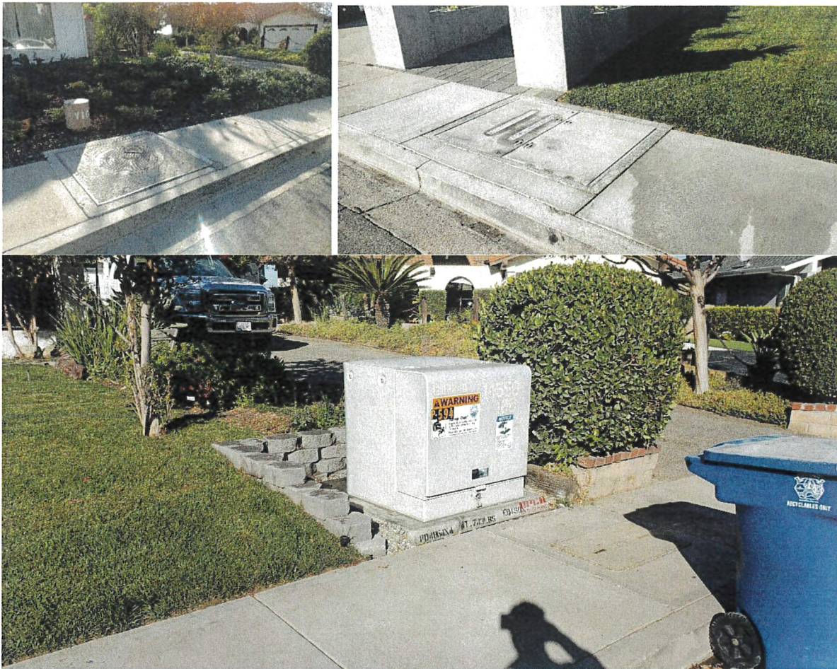
Vault 16 before and after
