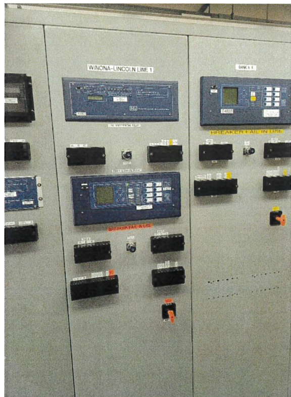
Post Replacement (new relays)
