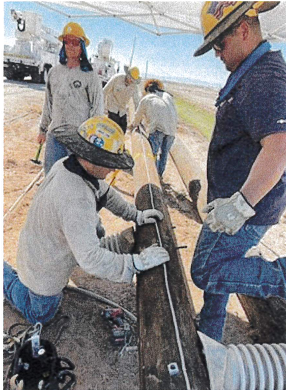
Figure 3 – BWP crew preparing a new pole prior to installation
