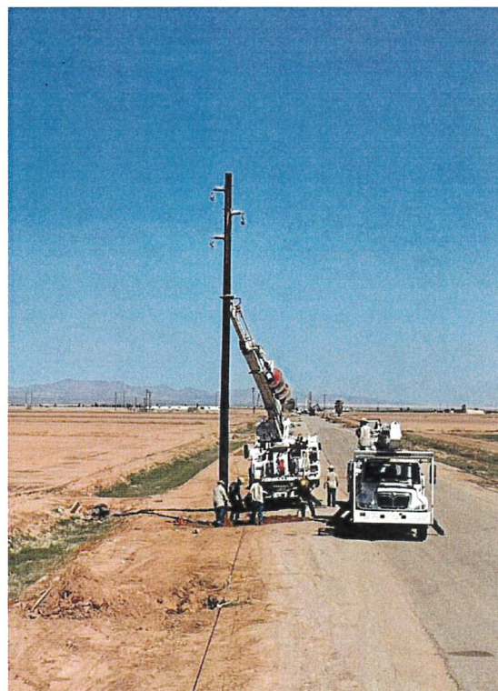
Figure 4 – BWP crew installing a new pole after clear-out of road
