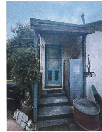
SIDE OF EXISTING RESIDENCE VIEW C
