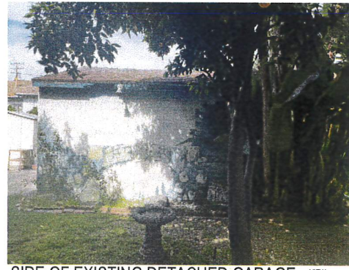
SIDE OF EXISTING DETACHED GARAGE VIEW D
