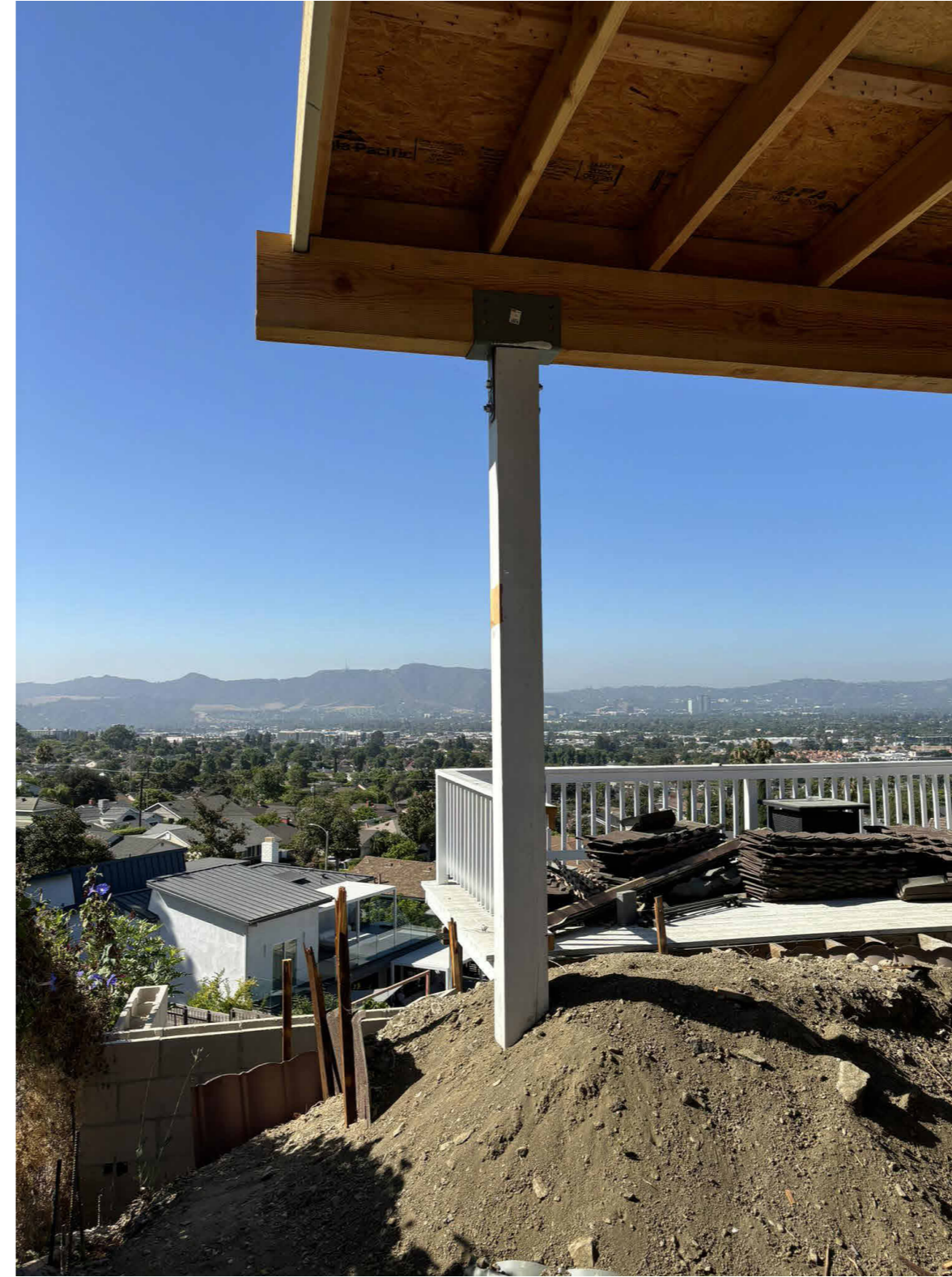
C - REAR OF THE PROPERTY
