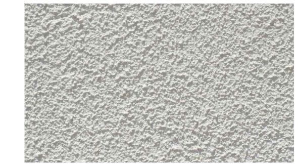
1 EXISTING WHITE SAND FINISH CEMENT PLASTER
