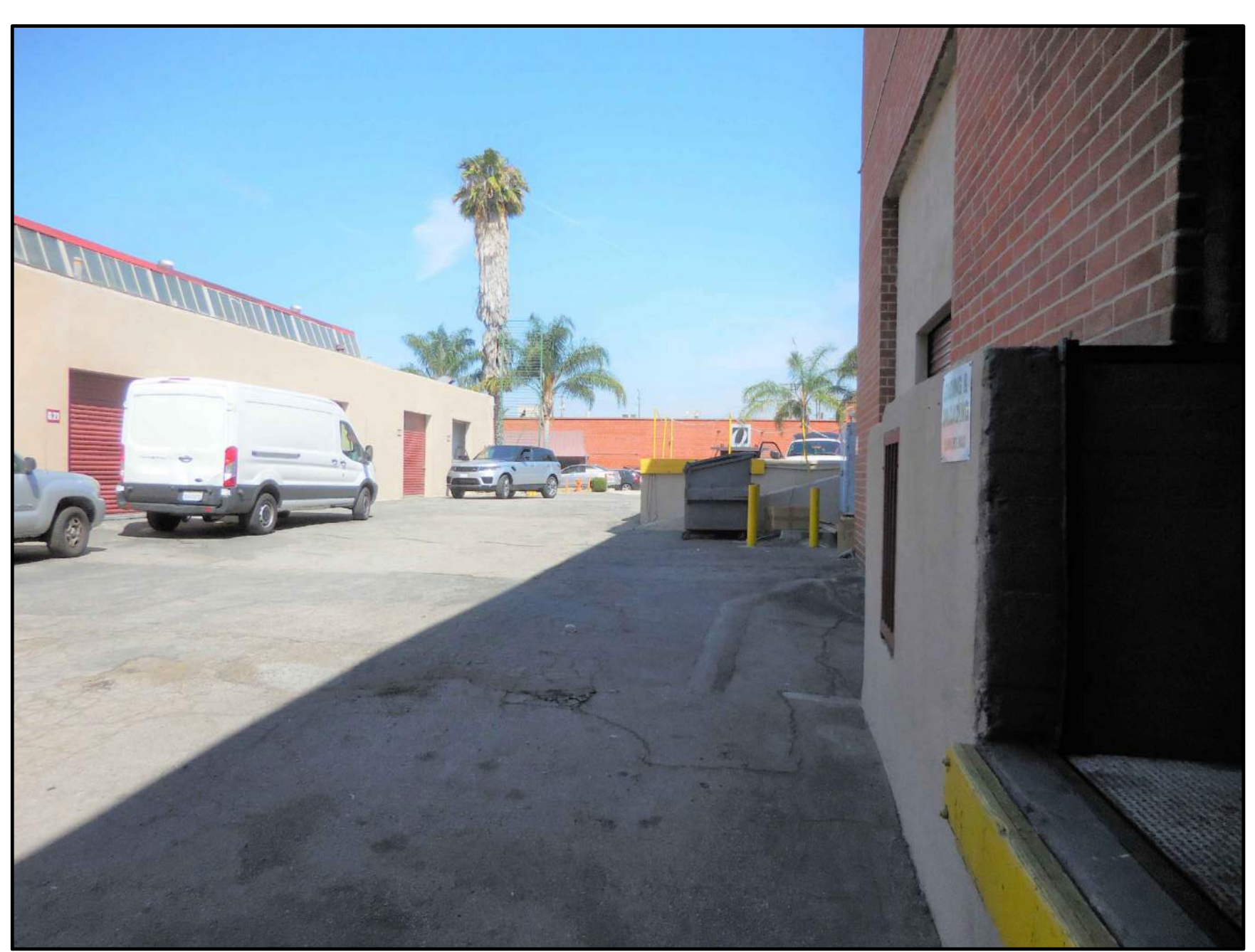
13 SOUTH DRIVE-WAY LOOKING AT WEST NORTH
