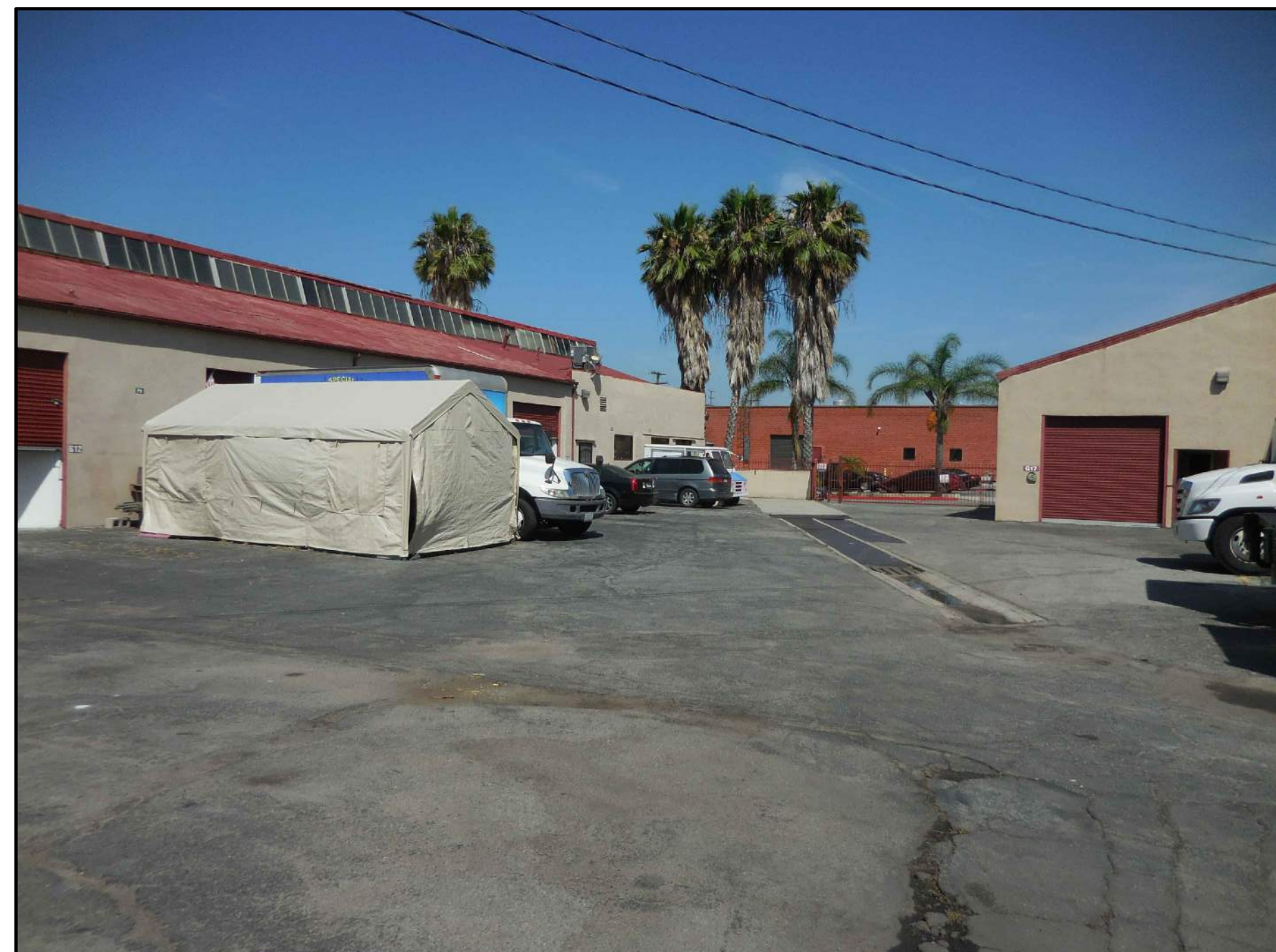
7 SOUTH DRIVE-WAY LOOKING AT NORTH WEST DRIVEWAY
