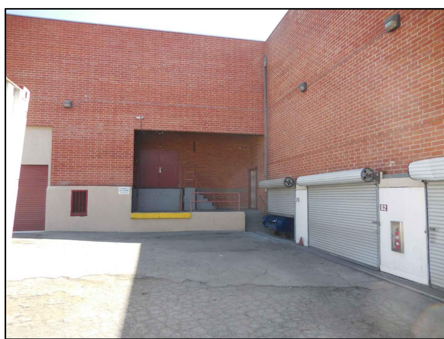
9 SOUTH DRIVE-WAY LOOKING AT SOUTH WEST DRIVEWAY
