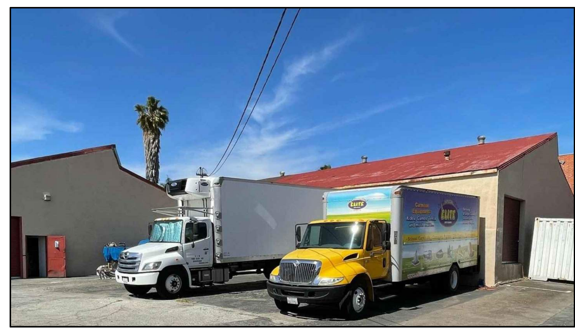
14 EXISTING BUILDING "A" LOOKING AT NORTH EAST
