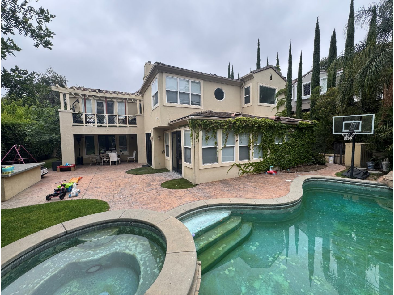
Figure 7d: Existing north elevation photo
