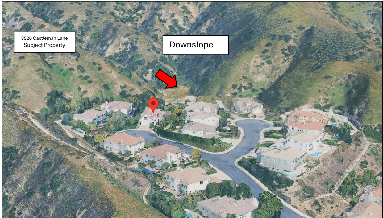
Figure 4a: Aerial photo of subject property
