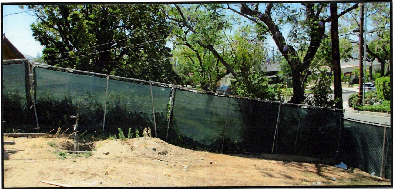
Figure 8: View of the proposed new retaining wall located in the front yard area with a proposed maximum height of 2'-6". The photo is looking southeast towards neighboring property 426 S. Sunset Canyon Drive.
