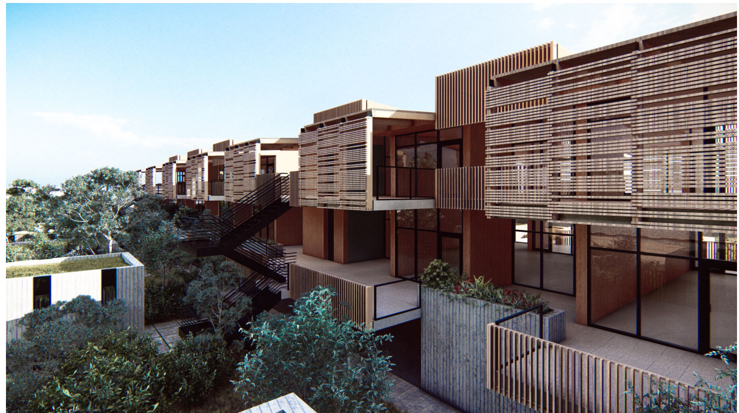
VIEW OF SOUTH FACADE - LOOKING NORTH WEST
