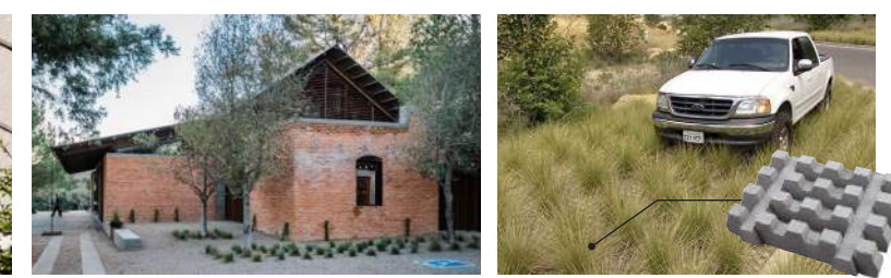
Turf Block concrete pavers, planted with grasses
