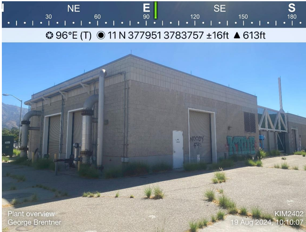
Photo 1. Overview of Plant on Eastern portion of project
