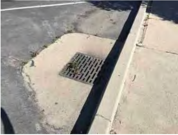
7. View of a typical storm water drain
