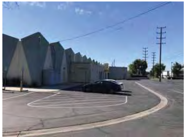
2. View of the western side of the subject property, facing south from the parking lot
