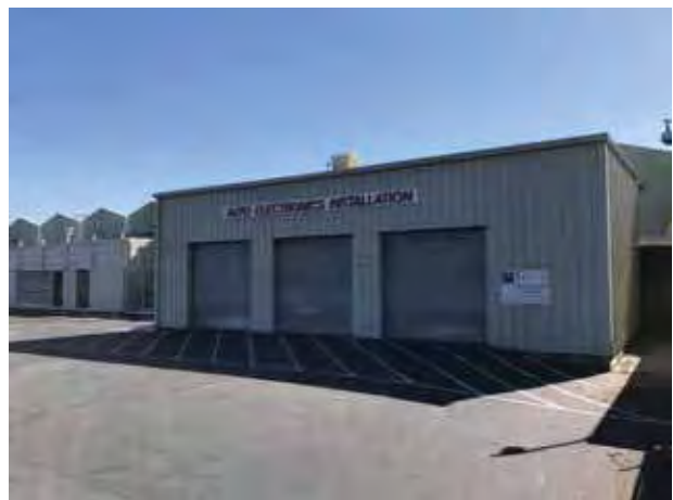
6. View of the inoperable automotive stereo installation garage
