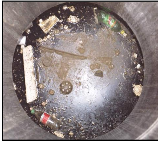
Floatable debris in the Aqua-Swirl®
