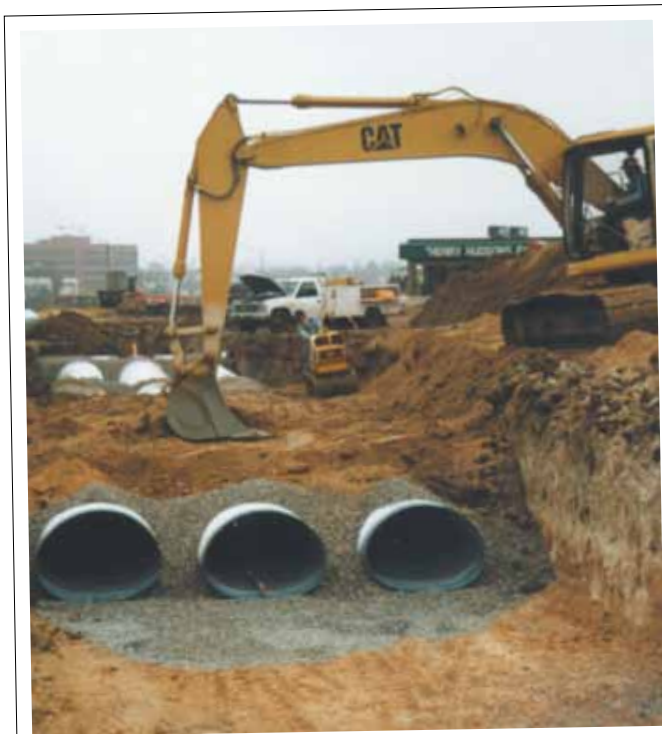
Pipe-arch for low profile application.
