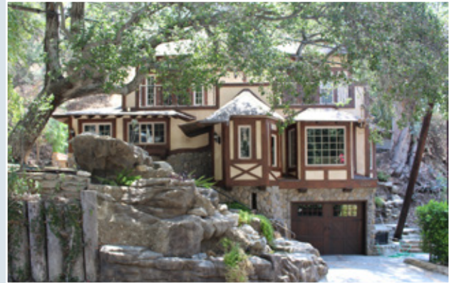
Figure 17 - The most visually fitting Hillside residences are cut into and/or follow the topography to reduce the perception of height and bulk and honor the natural settings.
