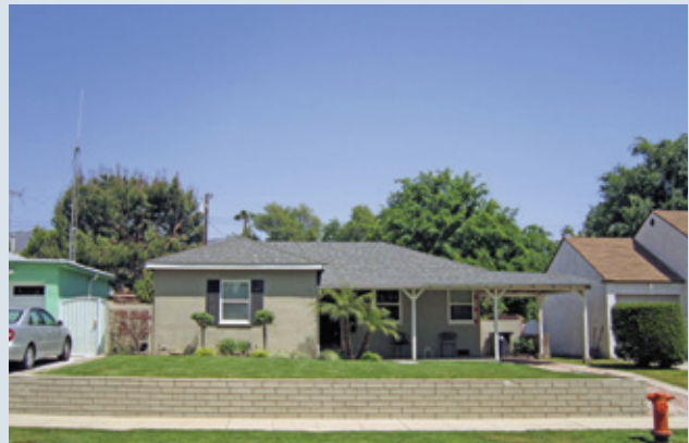
Figure 25 - A home with decorative shutters, and low pitched and hipped roofs, as well as minimal detailing exemplifies the Minimal Traditional/Colonial Revival style.
