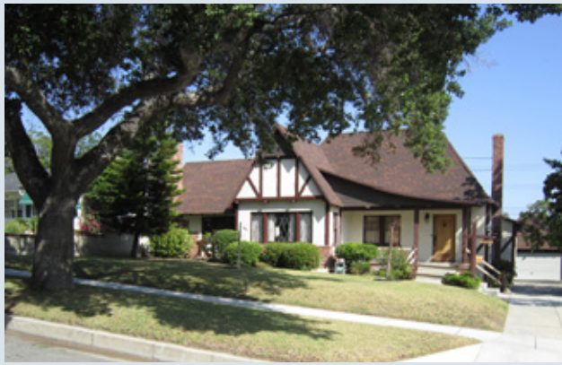
Figure 24 - A Tudor style home with diamond window panes, a board and batten entry door, and half-timbering. Note also the steeply pitched roofs and equilateral gable that faces the street that expresses the function of the main living area.
