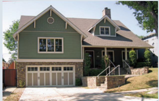
Figure 27 - This Split-Level home utilizes its parts to create a sense of more intimate scale. The garage is placed below the street-facing gabled form that features decorative roof brackets. In turn, this element, as well as the dormer over the recessed entry porch, create smaller masses that contrast with the overall bulk. The overall sense of size is further mitigated by the retreating slope of the main roof.
