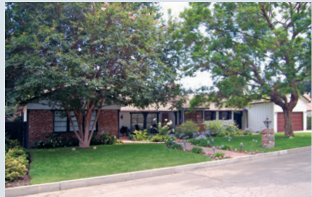
Figure 14 - In the Rancho, trees shade front lawns. In this residence, change in materials, from brick to vertical board and batten at the garage, and its separate small projecting mass, subordinate this latter volume in relationship to the horizontal length and breadth of the home. The entry, marked by the recess in the front wall plane, creates further visual interest.
