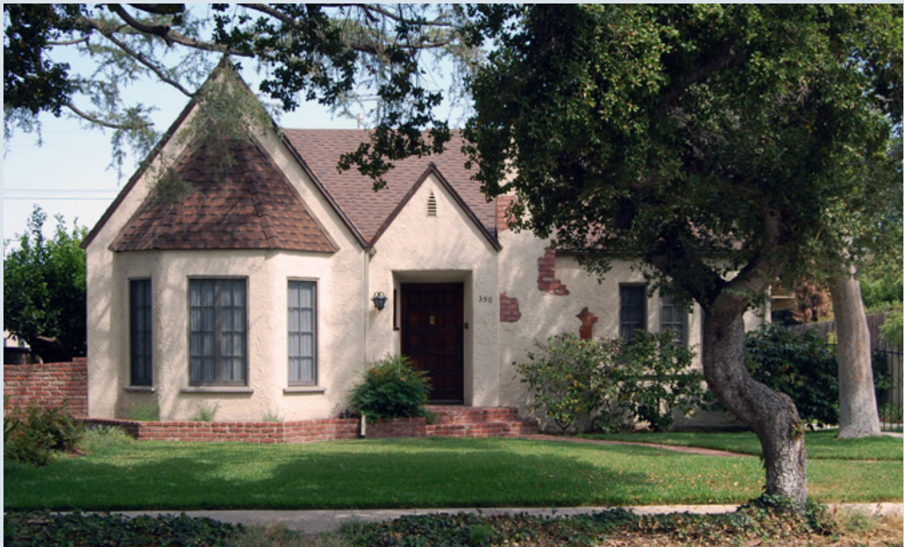
Figure 21 - This Tudor style home has steep roofs, expressed on the front façade by different sized equilateral-shaped gables. The roofed bay window contrasts with the vertical and narrow slot windows. The decorative brick and stucco chimney introduces additional visual variety and interest to this house.
