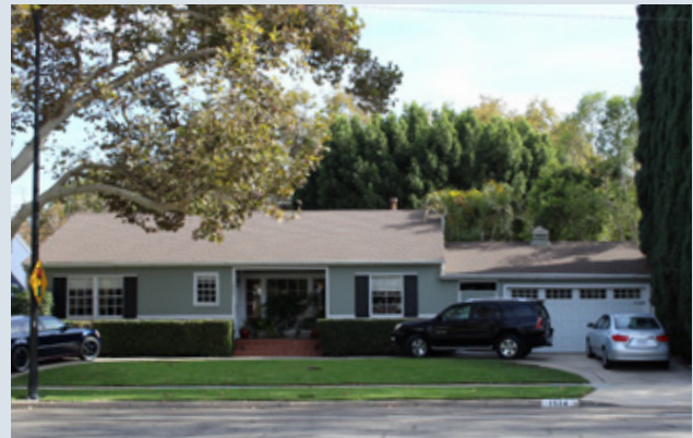
Figure 15 - The garage of this home is contiguous with the front of the main massing of the residence, but the lowered ridgeline subordinates its mass to the primary bulk of the dwelling.
