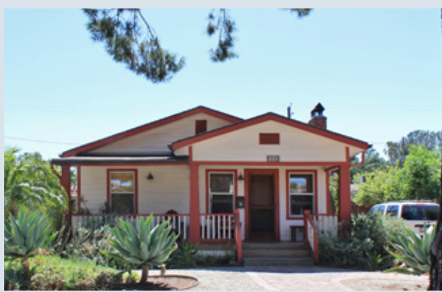
Figure 33 - Front entry placed within a secondary mass that is subordinate to and lower than the overall height of the building.
