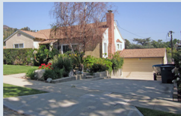
Figure 50 - Accessory structures and garages should be subordinate to the primary expression of the dwelling. In this home, the garage is set back from the front building plane and the placement downslope further reduces its bulk and impact on the appearance of the front yard and the public streetscape.
