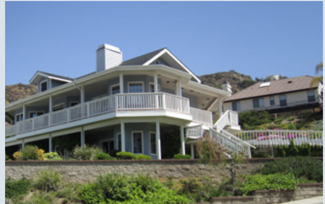
Figure 45 - The third story of this home is set under the pitch of the roof planes. The dormer at the third level adds visual interest to the home.
