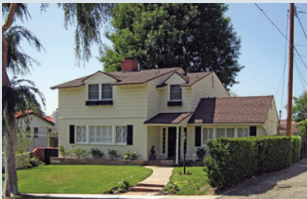
Figure 41 - Minor architectural components including dormers, planter boxes, three ridgelines at differing heights, a change of materials that distinguishes the second floor from the first floor, shutters, and a two-sided entrance porch and overhang each contribute to reducing the overall sense of bulk.
