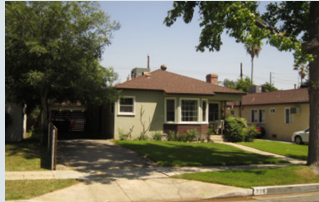
Figure 5 - Small single-family homes with garages placed to the rear of the lot characterize the Flats.
