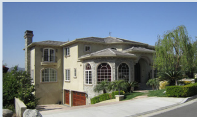
Figure 19 - This three-story home on a downslope lot follows the topography by having one story below street level, reducing the bulk and mass observed. Note the below-grade minimally visible garage.
