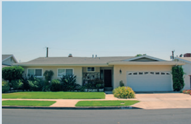
Figure 26 - The ground-hugging form of this one-story Ranch home is also echoed by the low-pitched, gabled and hipped and deep-eaved roof line.
