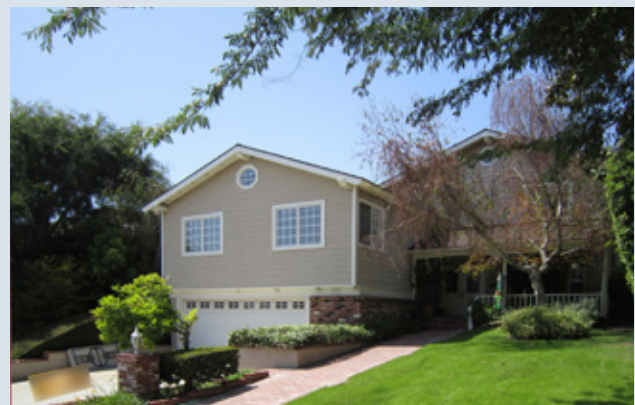
Figure 10 - Cut Hillside homes often deploy multi-ridged roofs at differing levels, reducing the bulk of the residence.
