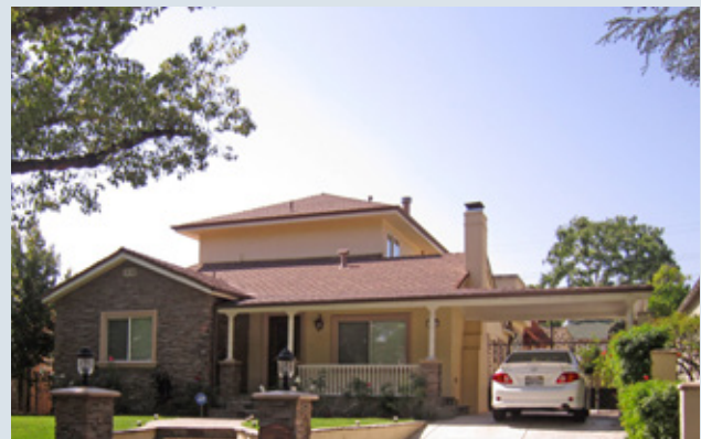
Figure 44 - Setting the mass of the second story behind the one-story roof ridgeline reduces the perception of bulk and maintains one-story character oriented towards the sidewalk.
