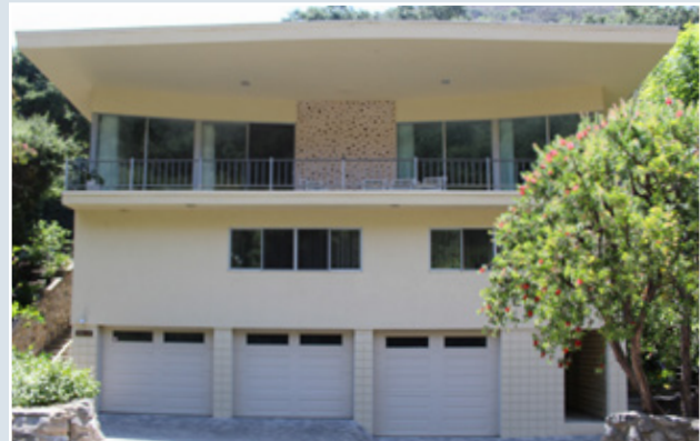
Figure 18 - Along some streets in the Hillside neighborhoods, irregular and topographically challenging sites lead to innovative expressions. Here the visual impact of the three-car garage is diminished by the character of the projecting roof, recess, and horizontal glass of the third level, creating a visual crown that leads the eye upward.
