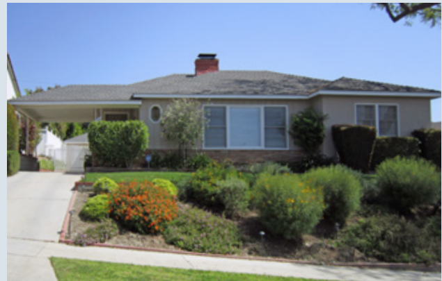
Figure 55 - Foundation plantings at the front façade create a natural transition from the lawn to the home. Low bushes and ground cover maintain views across the front yard, reduce the area of the traditional turf lawn, and save water.
