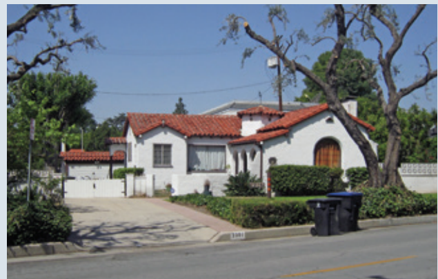
Figure 56 - Low hedges at the back of sidewalk, low walls at the entry, foundation plantings, and a traditional turf lawn maintain the appearance and character of this home.
