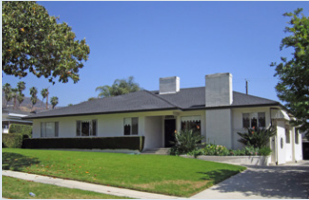
Figure 39 - The bulk of this home, under a uniform-in-height ridgeline, is articulated by a major mass that incorporates a recessed corner entry, and a minor asymmetric mass, accented by a vertical chimney.
