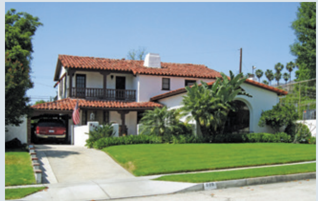
Figure 23 - Asymmetric massing and a forward-thrusting but subordinate living room mass characterize this Spanish Revival dwelling. The 1:3 roof pitch pierced by a trapezoidal chimney, use of red roof tile and light colored stucco, recessed front entry, and low-walled forecourt are all typical of the style.
