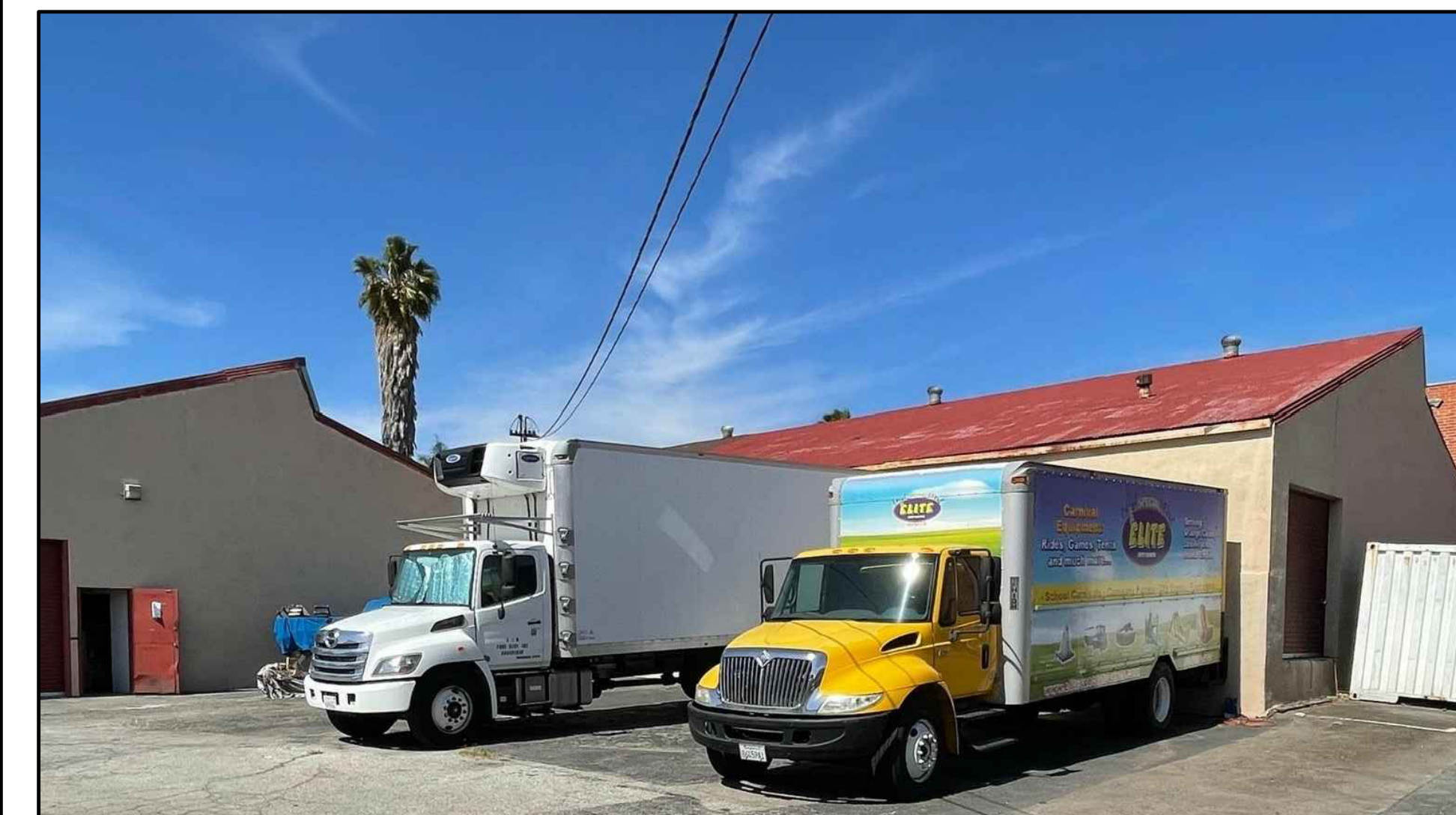
14 EXISTING BUILDING "A" LOOKING AT NORTH EAST
