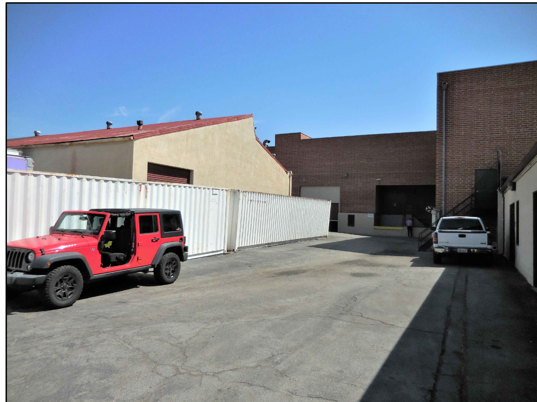
12 SOUTH DRIVE-WAY LOOKING AT NORTH EAST
