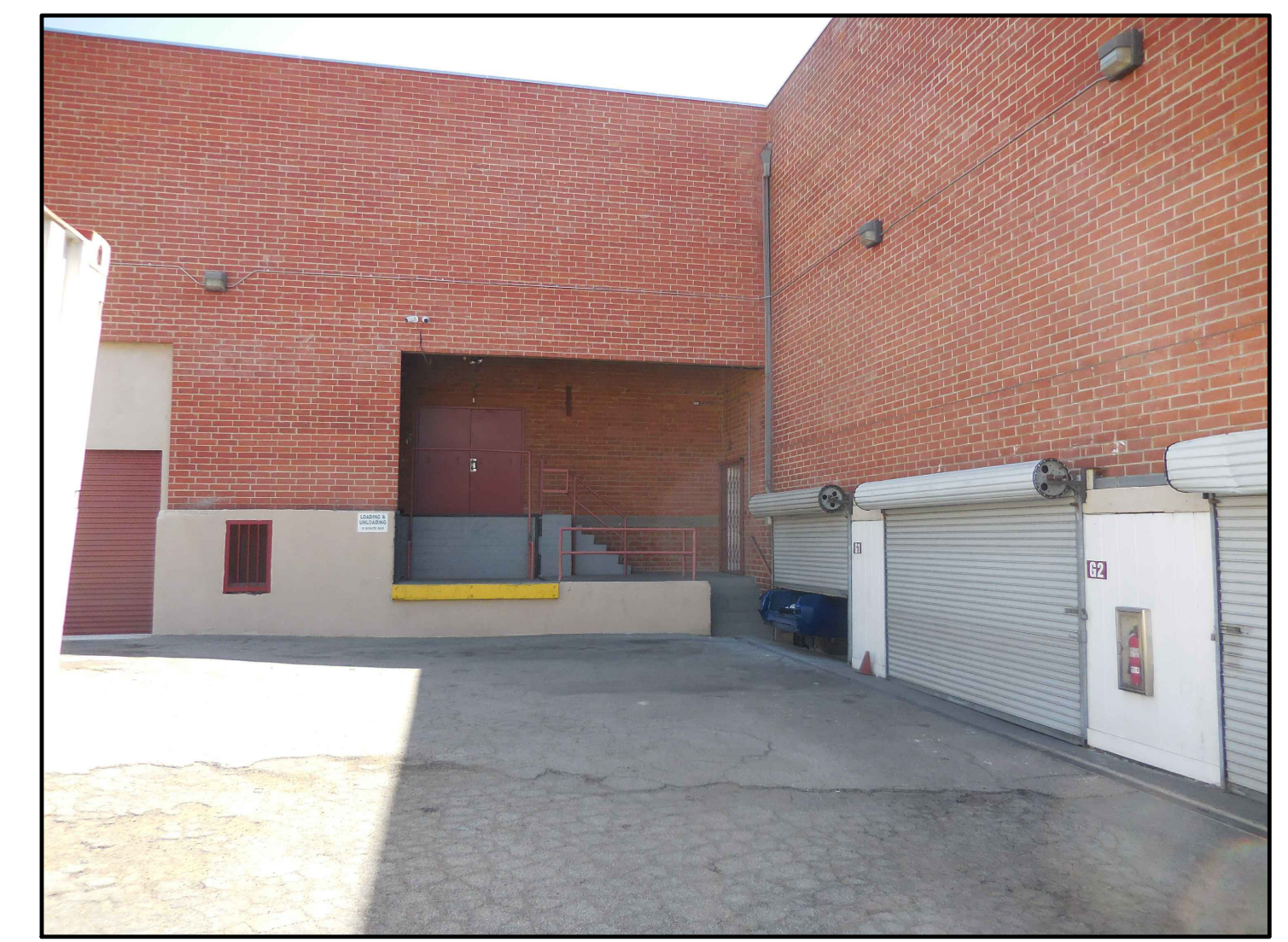
9 SOUTH DRIVE-WAY LOOKING AT SOUTH WEST DRIVEWAY
