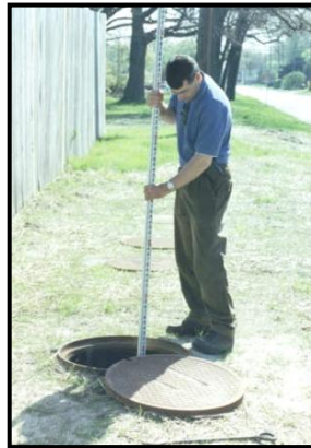
Sediment inspection using a stadia rod in a single chamber
