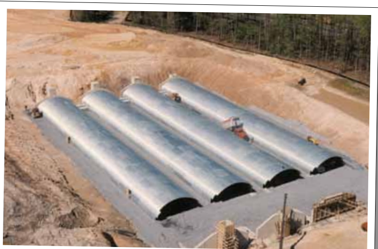
Plate system for high volume storage
