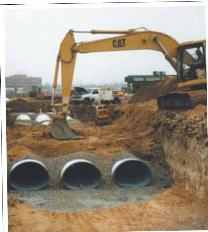
Pipe-arch for low profile application.
