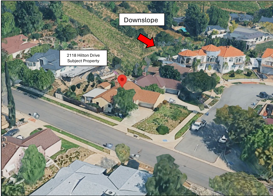
Figure 4a: Image of subject property looking northeast
