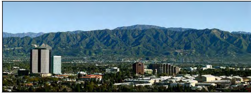
Steep slopes, such as those in the Verdugo Mountains in the northern part of Burbank, are subject to landslide hazards.
