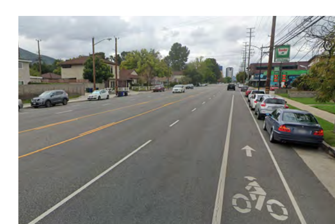
Alameda Ave - Existing
