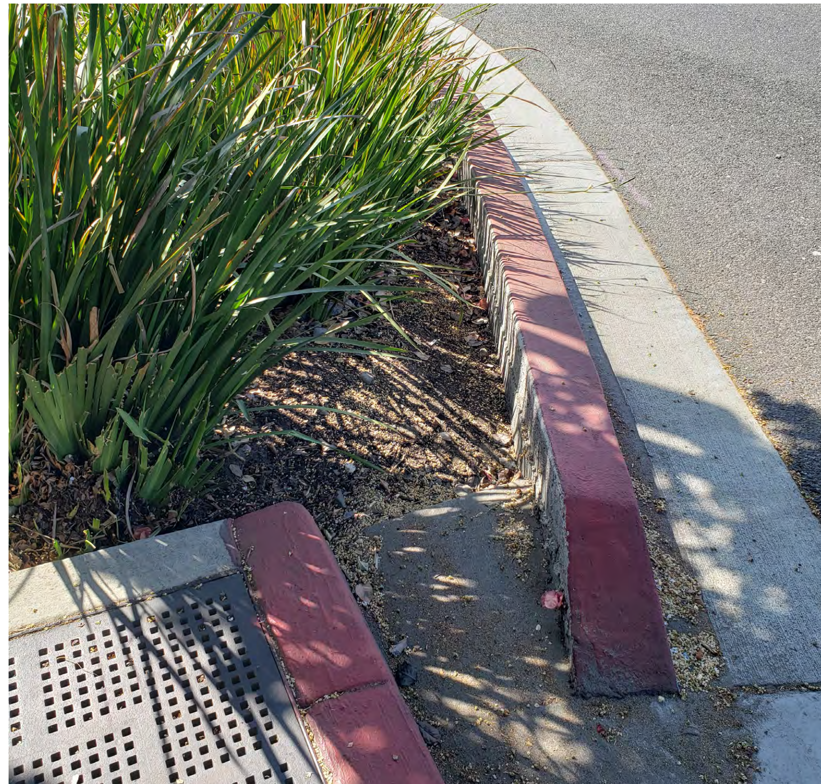
infiltration planters, lake street, burbank
