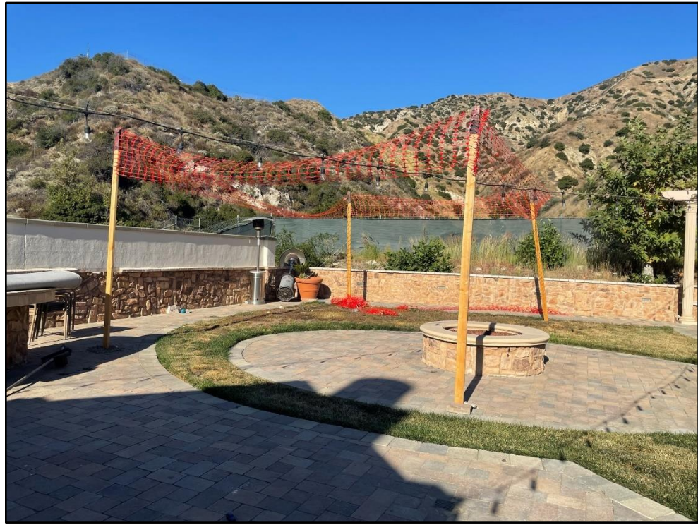
View of story pole installation located in the rear yard area of the subject property.
