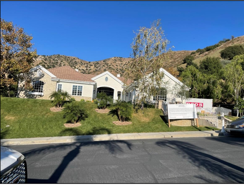
View from across Wedgewood Lane of the subject property.
