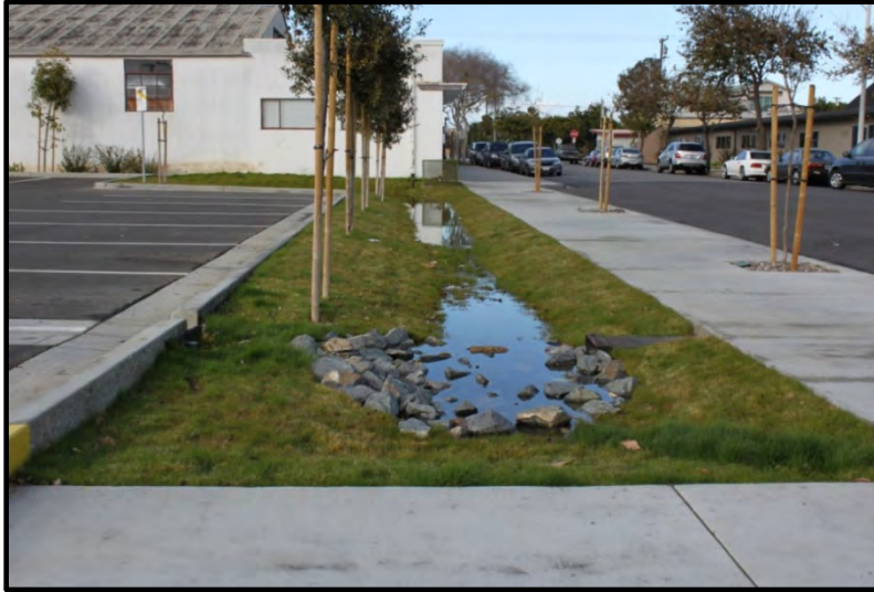
Figure 8: Vegetated swale (Signal Hill, CA).
