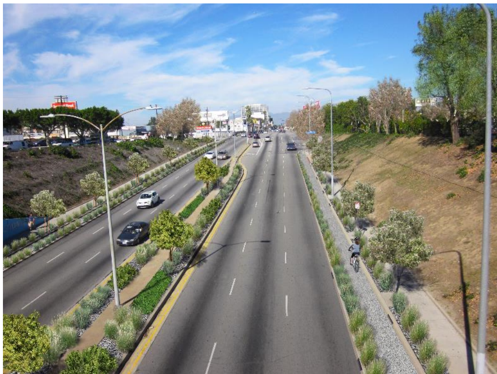
Figure 27. Conceptual rendering showing protected bike lane with permeable pavement and bioretention.
