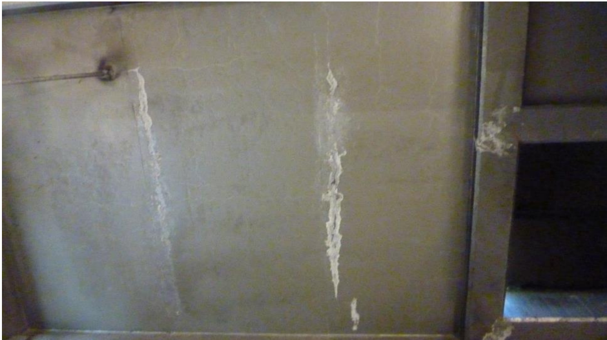
Figure 7. Roof Slab Cracks Adjacent to Steel Roof Access Hatch.
