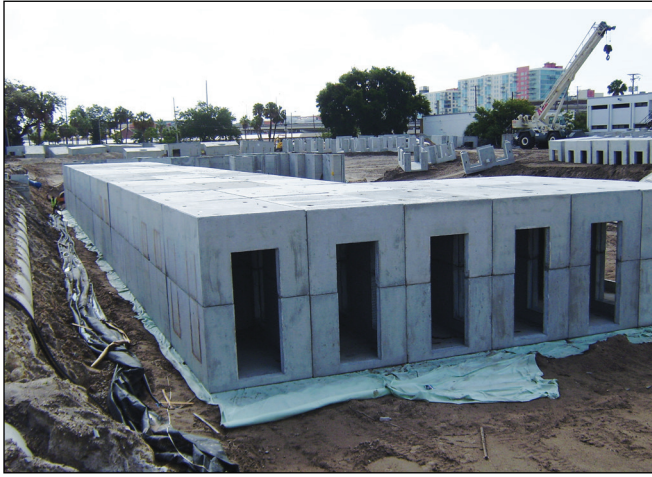
Same day staging and installation of StormCapture project.
