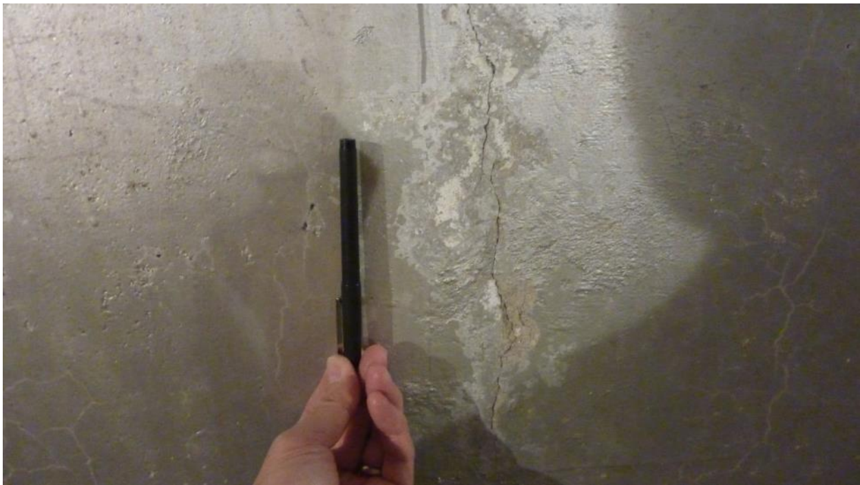
Figure 11. Close-up View of Vertical Wall Crack.
