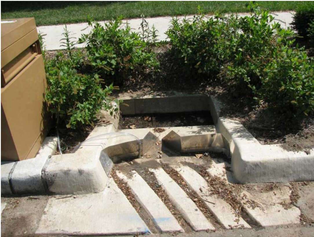
Figure 29. Inlet curb cut with an H-flume.
