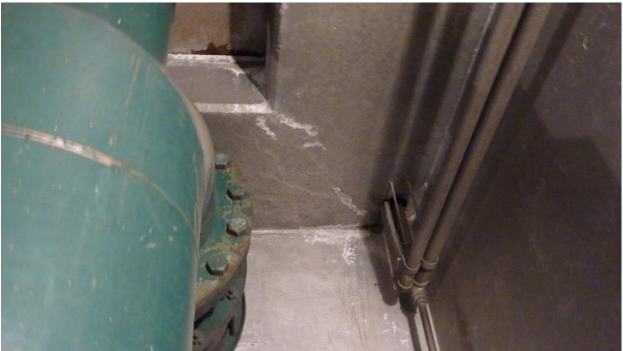
Figure 9. Cracks at Bottom of Motor Room Floor Slab Opening.
