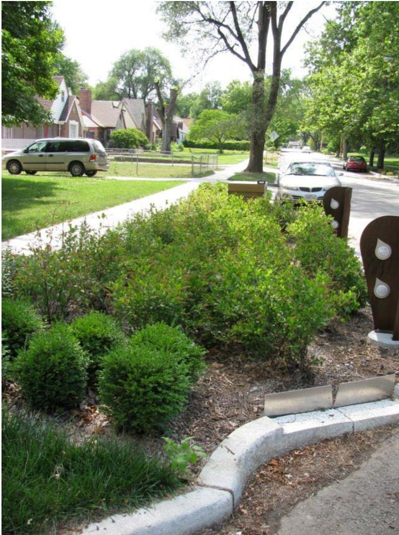
Figure 30. Outlet of a roadside bioretention equipped with a V-notch weir for flow monitoring.
