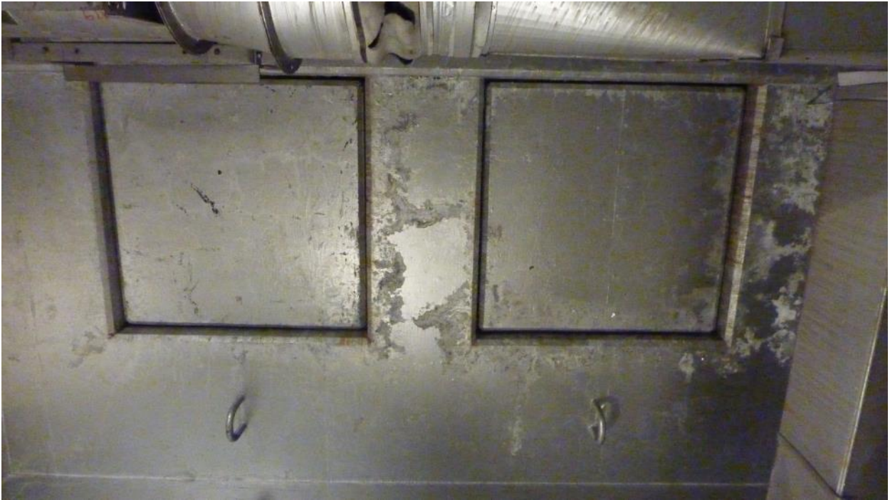
Figure 8. Roof Beam Cracks with Water Stains at Concrete Roof Hatches.
