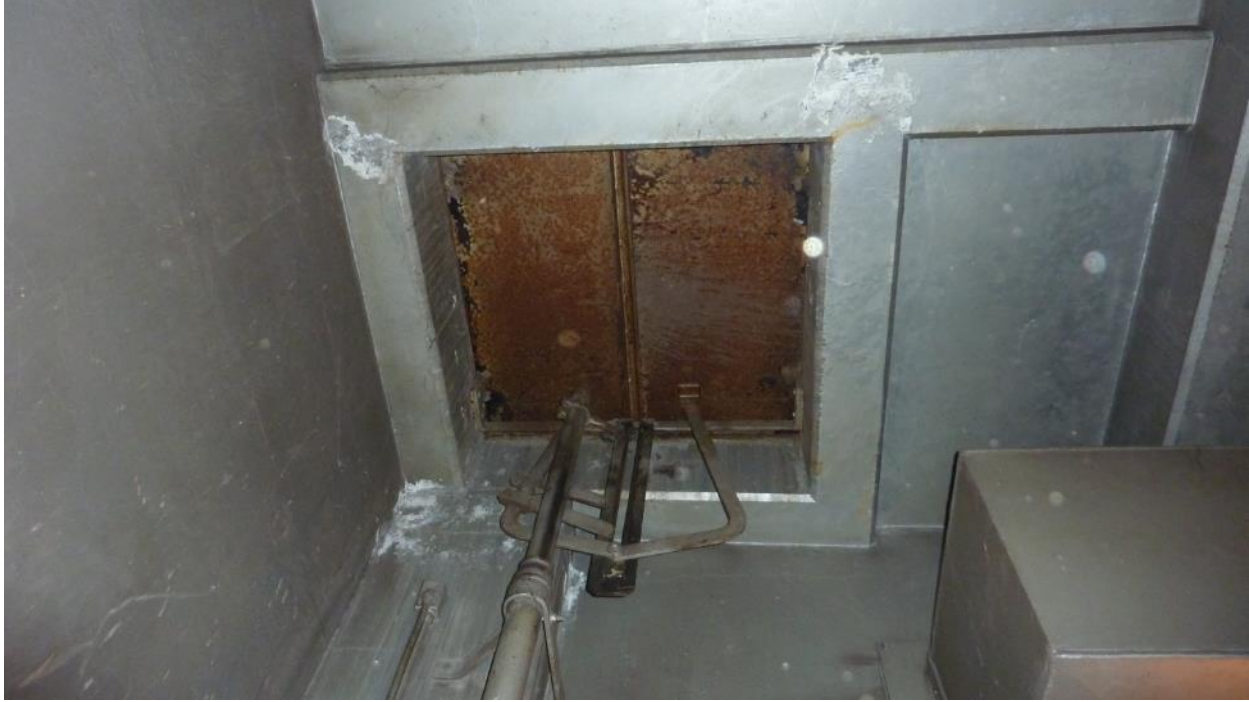
Figure 6. Surface Corrosion at Steel Access Hatch Cover and Roof Beam Cracks with Water Stains.
