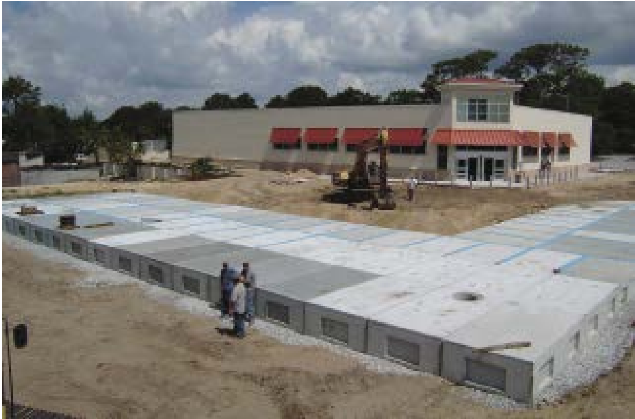
Figure 21. Subsurface Infiltration Gallery. (Source: www.oldcastlestormwater.com )
