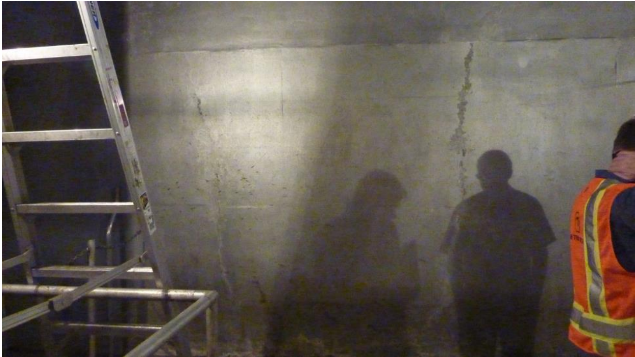
Figure 10. Vertical Wall Cracks in East Wall of Bar Screen Room (left of center and right of center).
