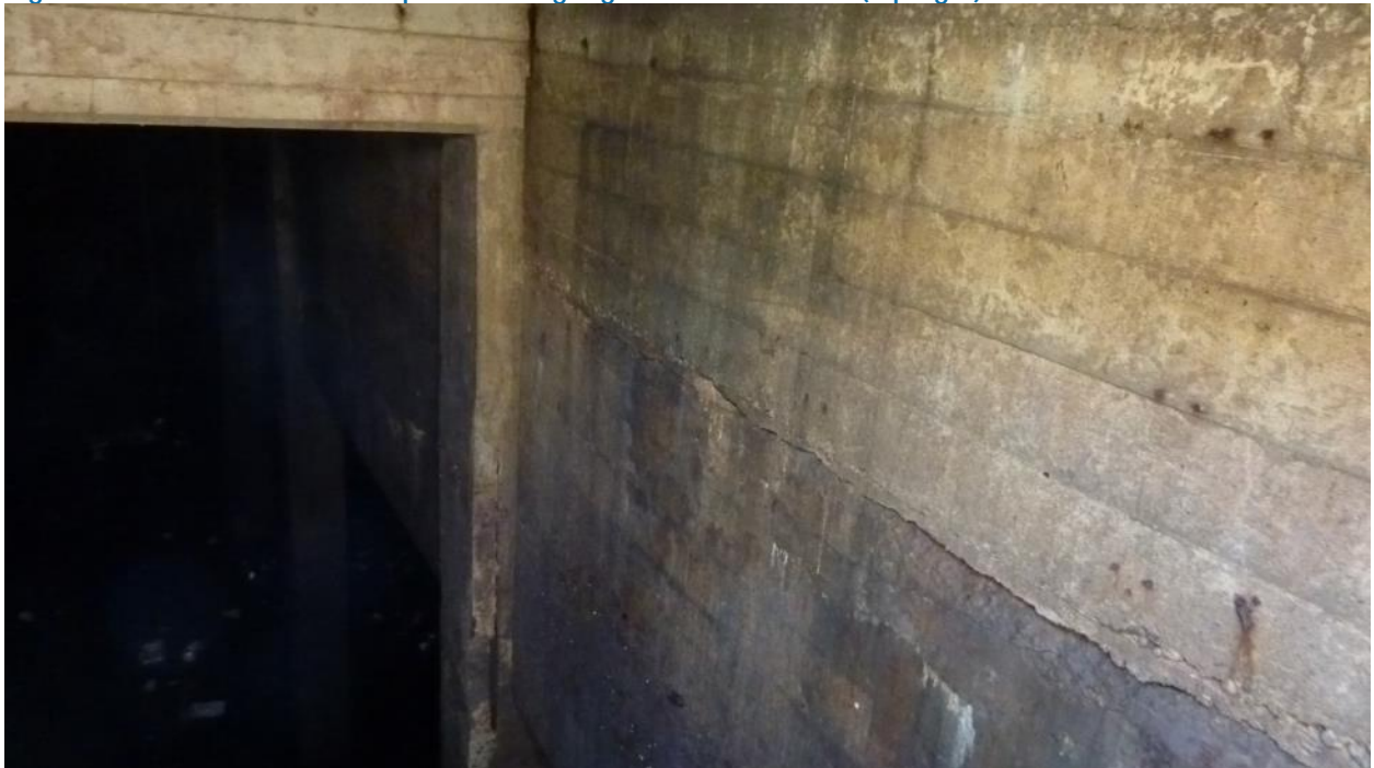
Figure 10. Surge Chamber Support Column Concrete Spall (bottom) and Wall Crack (middle).
