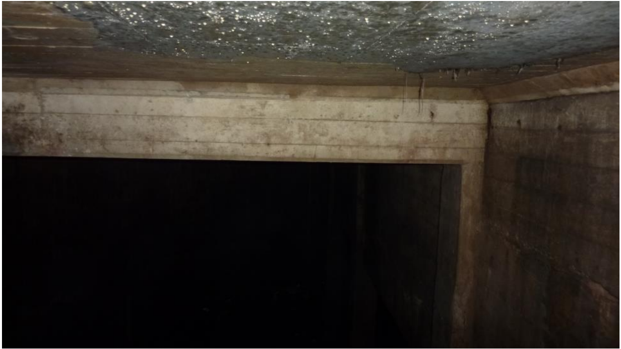
Figure 9. Wet Well Roof Slab Repair Showing Signs of Delamination (top right).
