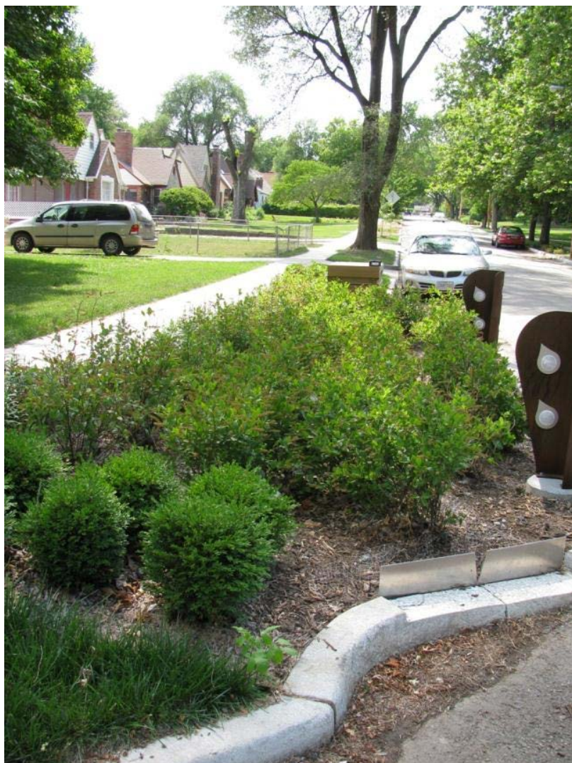
Figure 29. Outlet of a roadside bioretention equipped with a V-notch weir for flow monitoring.
