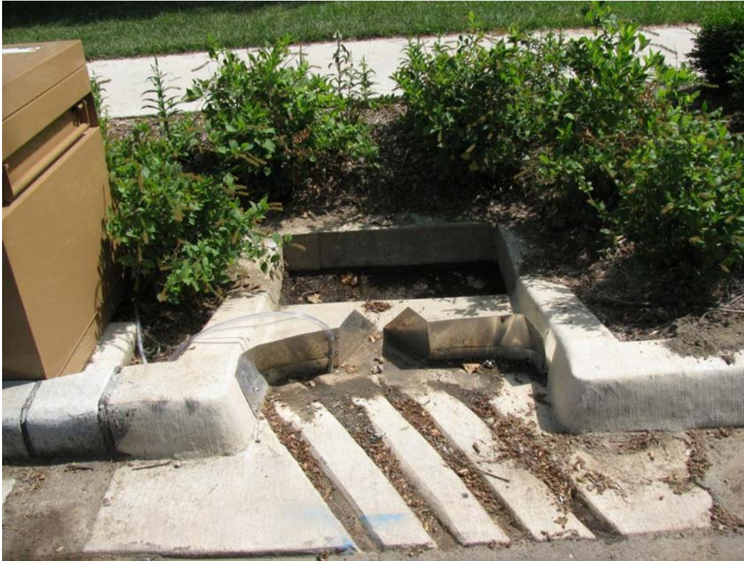
Figure 22. Inlet curb cut with an H-flume.
