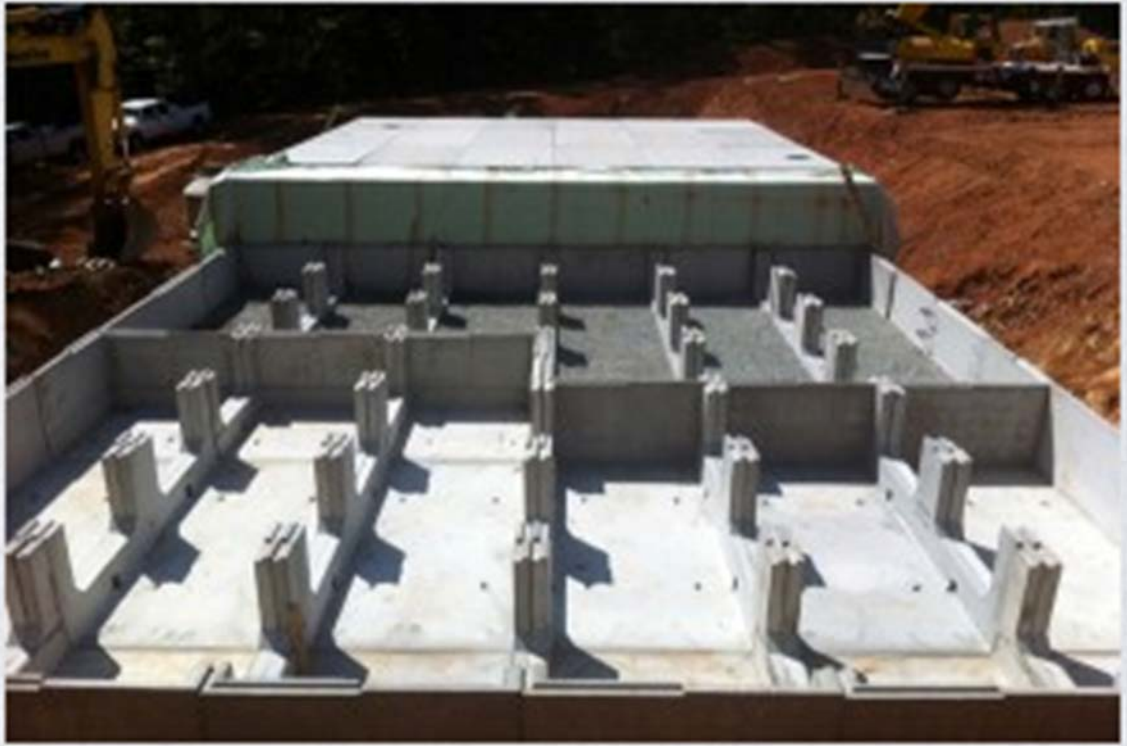
Figure 21. Subsurface Storage Gallery. (Source: www.oldcastlestormwater.com )
