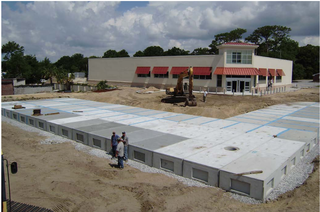
Figure 15. Subsurface Infiltration Gallery. (Source: www.oldcastlestormwater.com )
