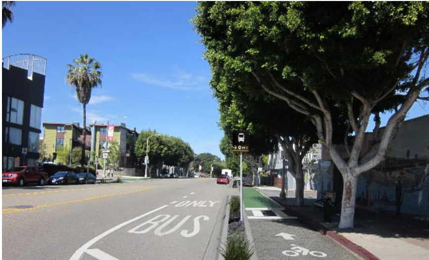
Figure 26. Conceptual rendering showing protected bike lane with permeable pavement and bioretention.
