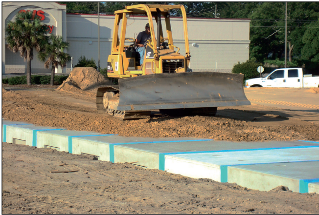
StormCapture modules are designed for HS20 traffic loading.
