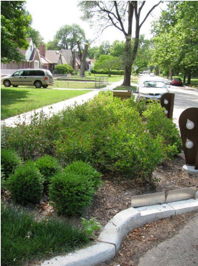
Figure 23. Outlet of a roadside bioretention equipped with a V-notch weir for flow monitoring.
