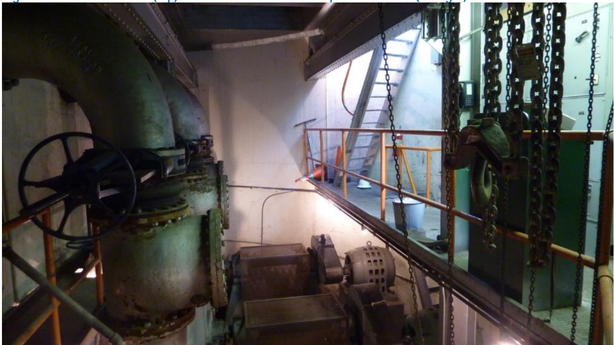
Figure 8. Aisle Between Ships Ladder and Guardrail is Substandard (middle) and Obstructed.
