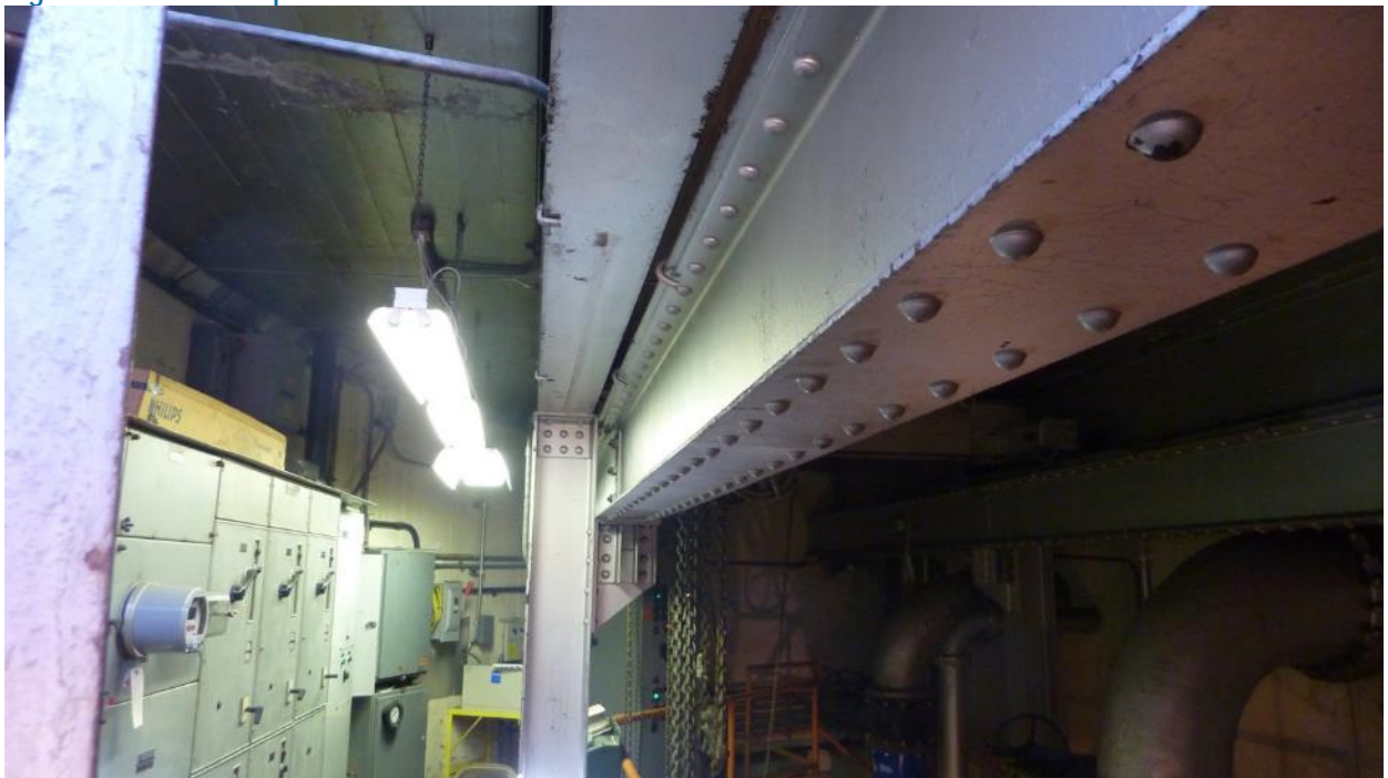
Figure 6. Roof Slab Crack (upper left) Over Electrical Panels.
