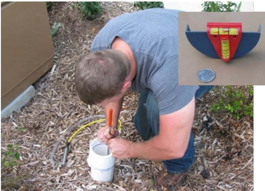
Figure 24. Typical weir for monitoring flow in an underdrain.
