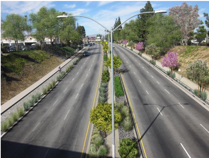
Figure 20. Conceptual rendering showing protected bike lane with permeable pavement and bioretention (Note: BMPs are not recommended in the median. Vegetation in the median is a component of the Great Streets Initiative referenced in Section 4.).
