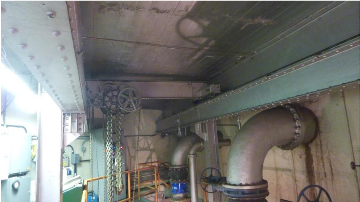
Figure 7. Roof Slab Crack (top) and Water Stains Under Pipe Penetration (far right).
