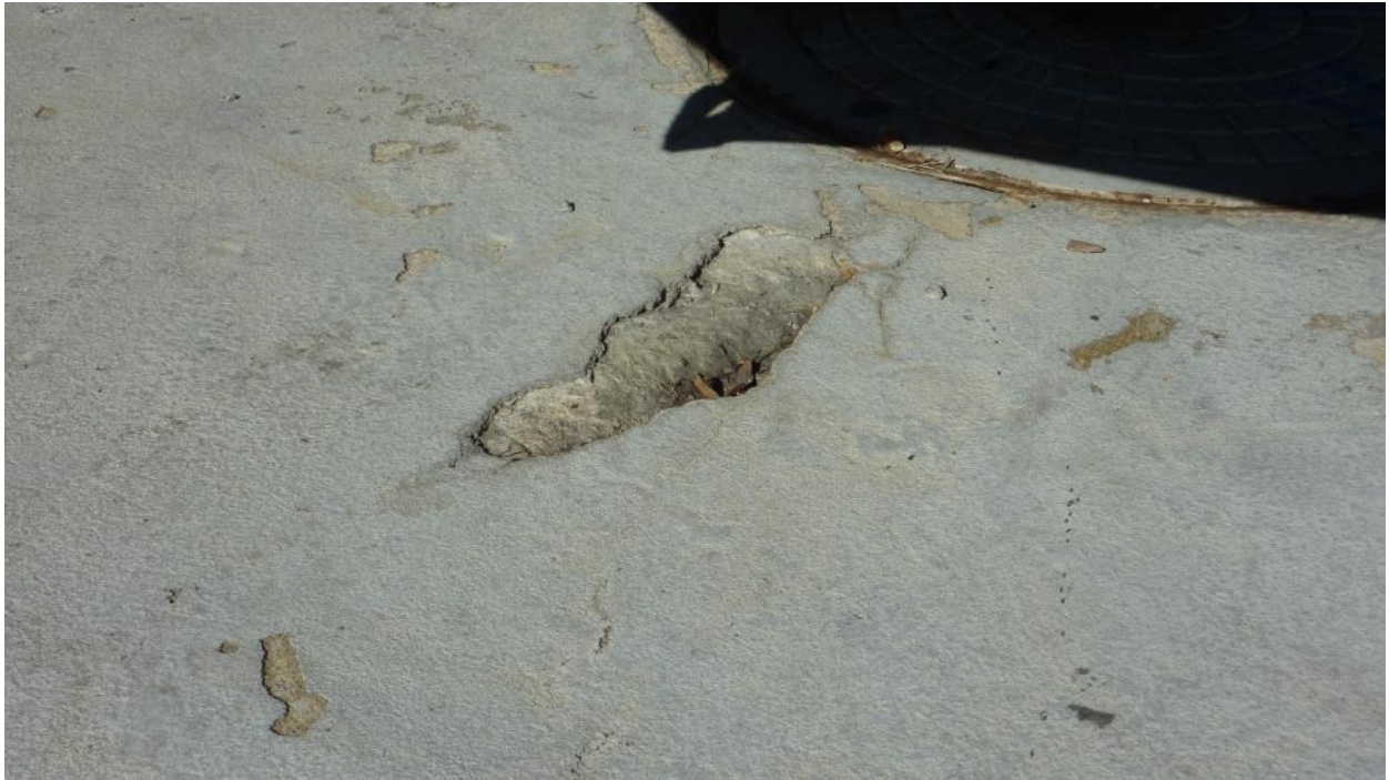
Figure 5. Roof Slab Spall.
