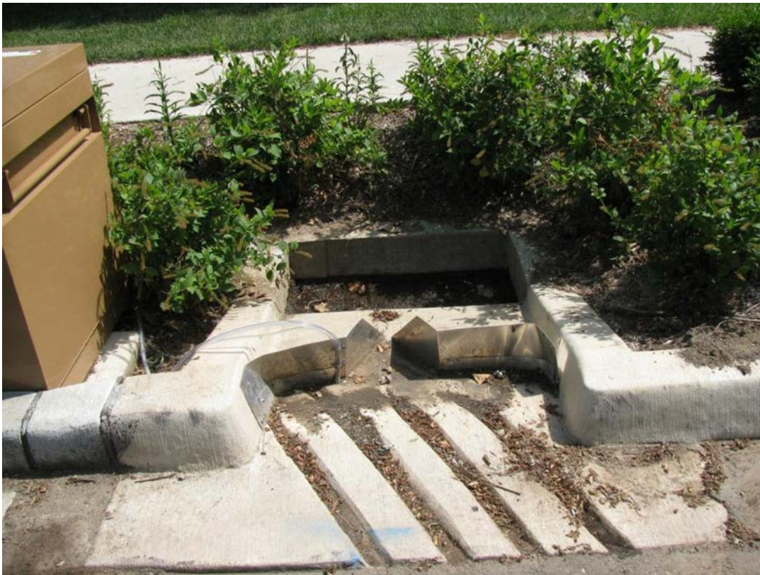
Figure 28. Inlet curb cut with an H-flume.
