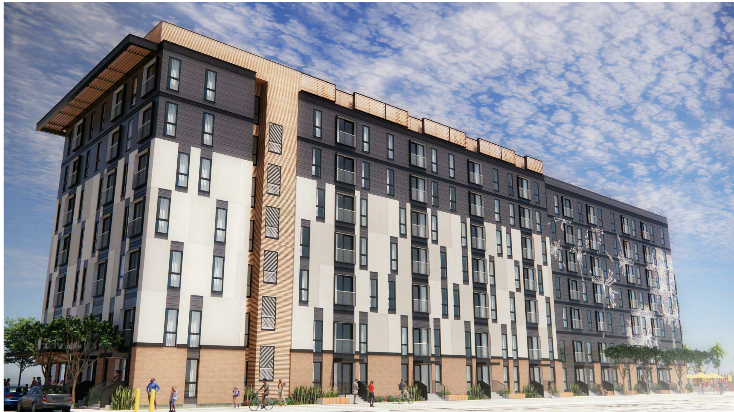
VIEW OF NORTH-WEST CORNER
