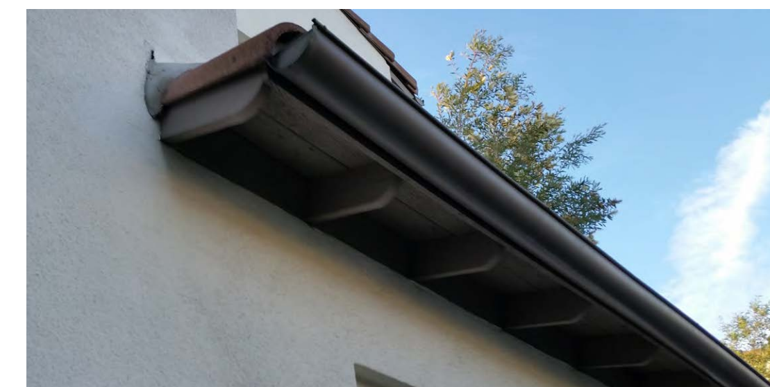
P. Exposed Wood Truss Tails with 2x3 Wood Fascia
