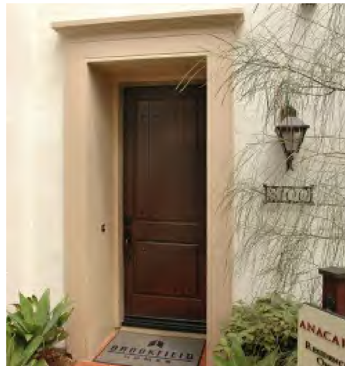
D. Stucco Entry Surround
