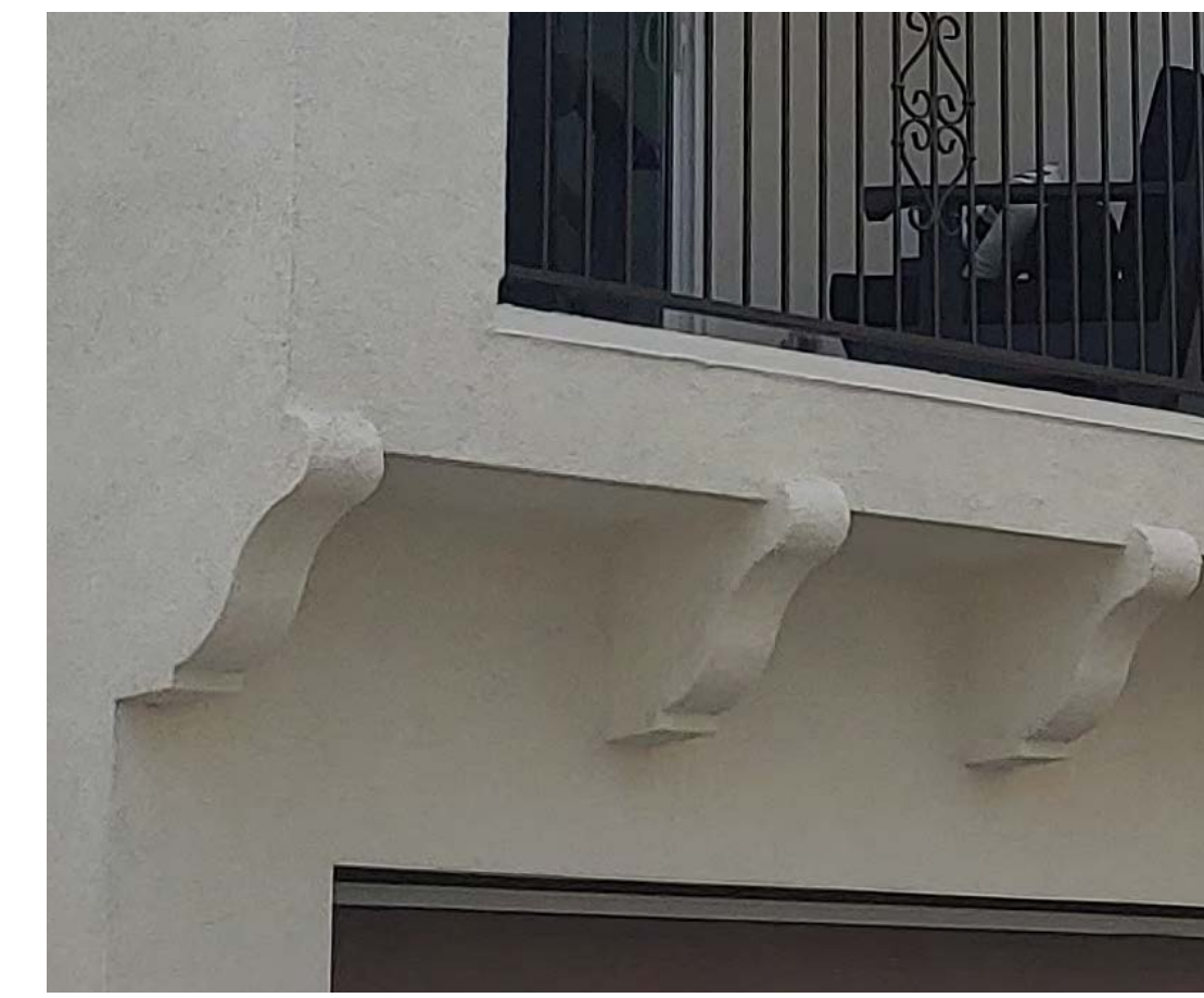
N. Decorative Stucco Corbels at Cantilever
