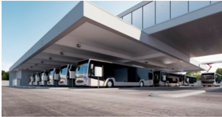
Figure 1-3: Buses Parked in Lanes Example (Source: ABB)
