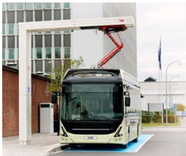
Figure 1-8: On-route Overhead Charging (Source: ABB)
