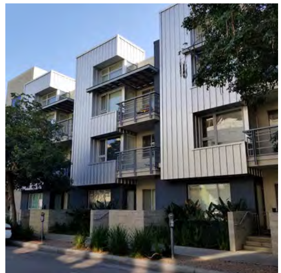
Walls along street-facing frontage of a ground floor residential unit
