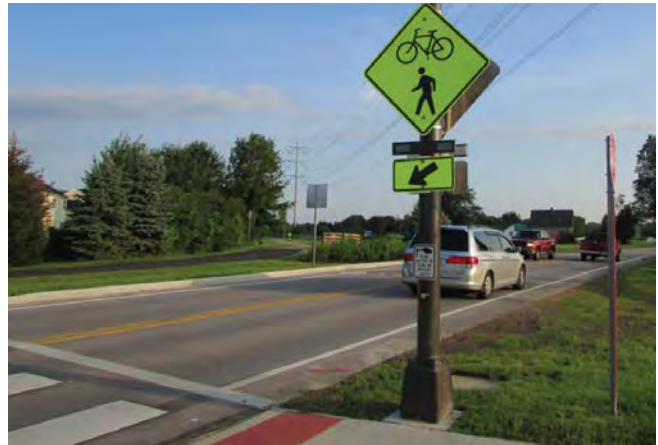
Rectangular Rapid Flashing Beacon (FHA)
