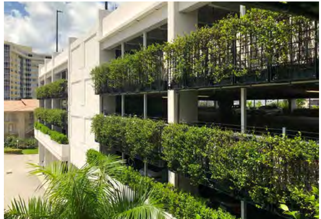
Landscaped parking structure facade
