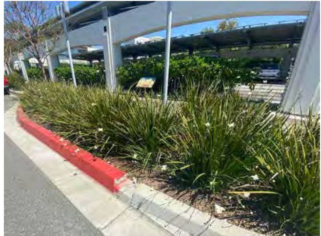
Bioswale curb extension
