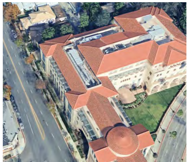
Roof-mounted equipment screened by parapet
