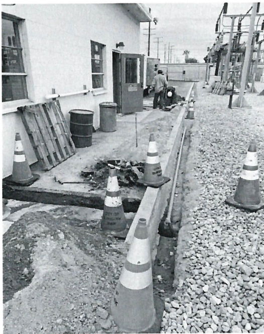
Valley Station Safety Shower (During Construction)
