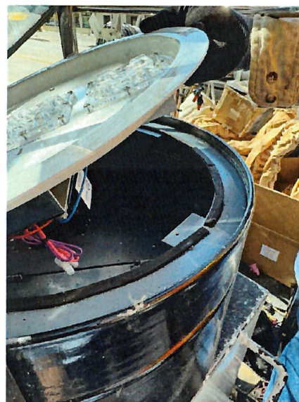
3-Ring Halo LED Conversion in Progress
