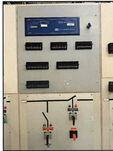
New Microprocessor Bus Relays @ Keystone
