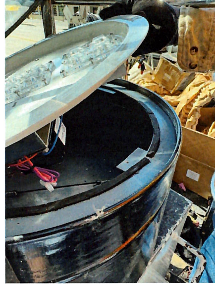
3-Ring Halo LED Conversion in Progress
