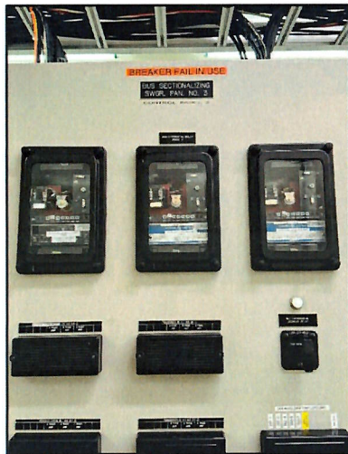
Older Electromechanical Bus Relays @Keystone
