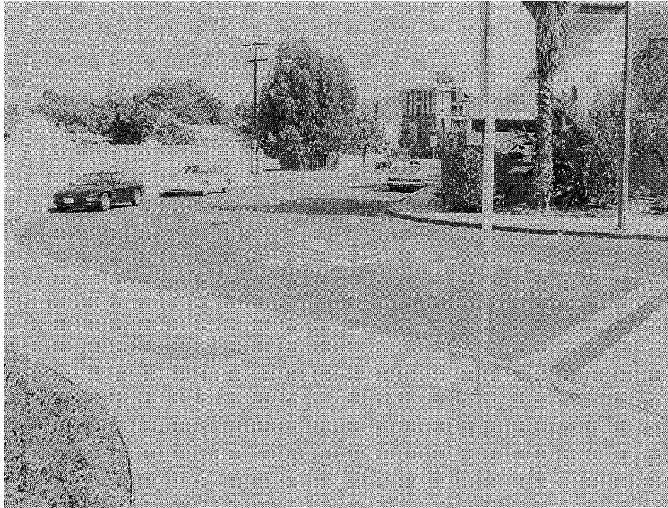
Realignment of Edison Road at Buena Vista Street
