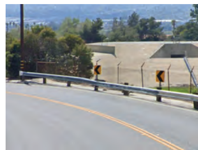
Curve Warning Signage
