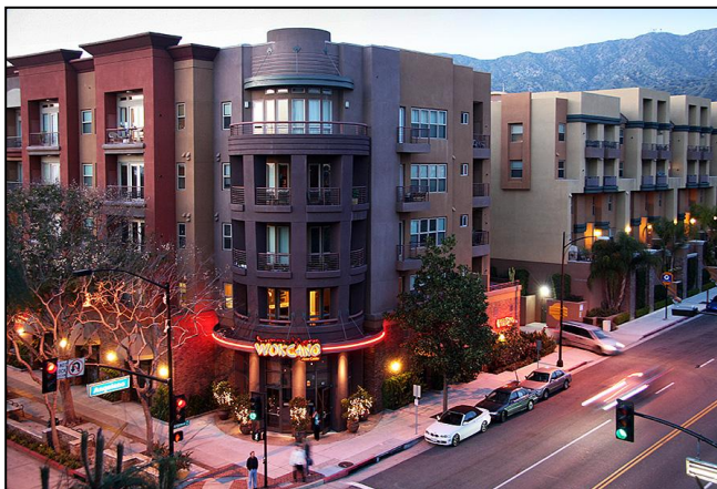
Mixed-use development contributes to a thriving community, but can place sensitive receptors adjacent to noisy businesses.
